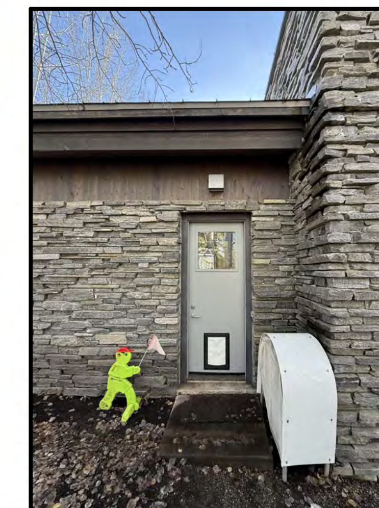
EXTERIOR LIGHT B LIGHT TYPE - EXISTING EXTERIOR DOOR DOWN LIGHT DARK SKY COMPLIANT
