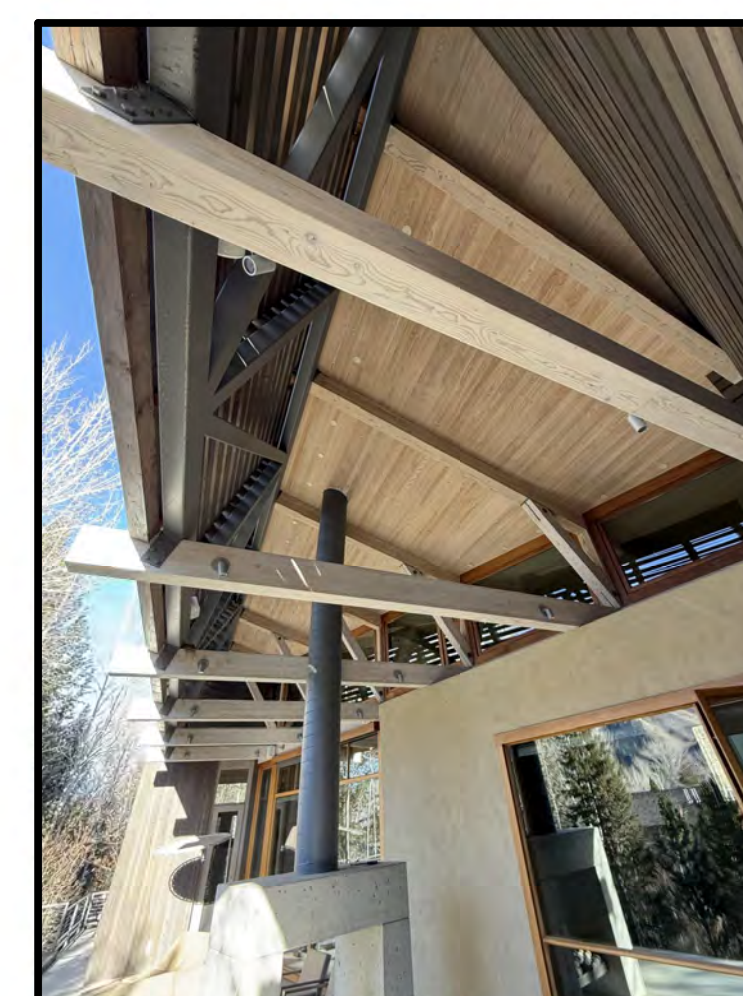
EXTERIOR LIGHT C LIGHT TYPE - EXISTING EXTERIOR PATIO DOWN LIGHTS DARK SKY COMPLIANT
