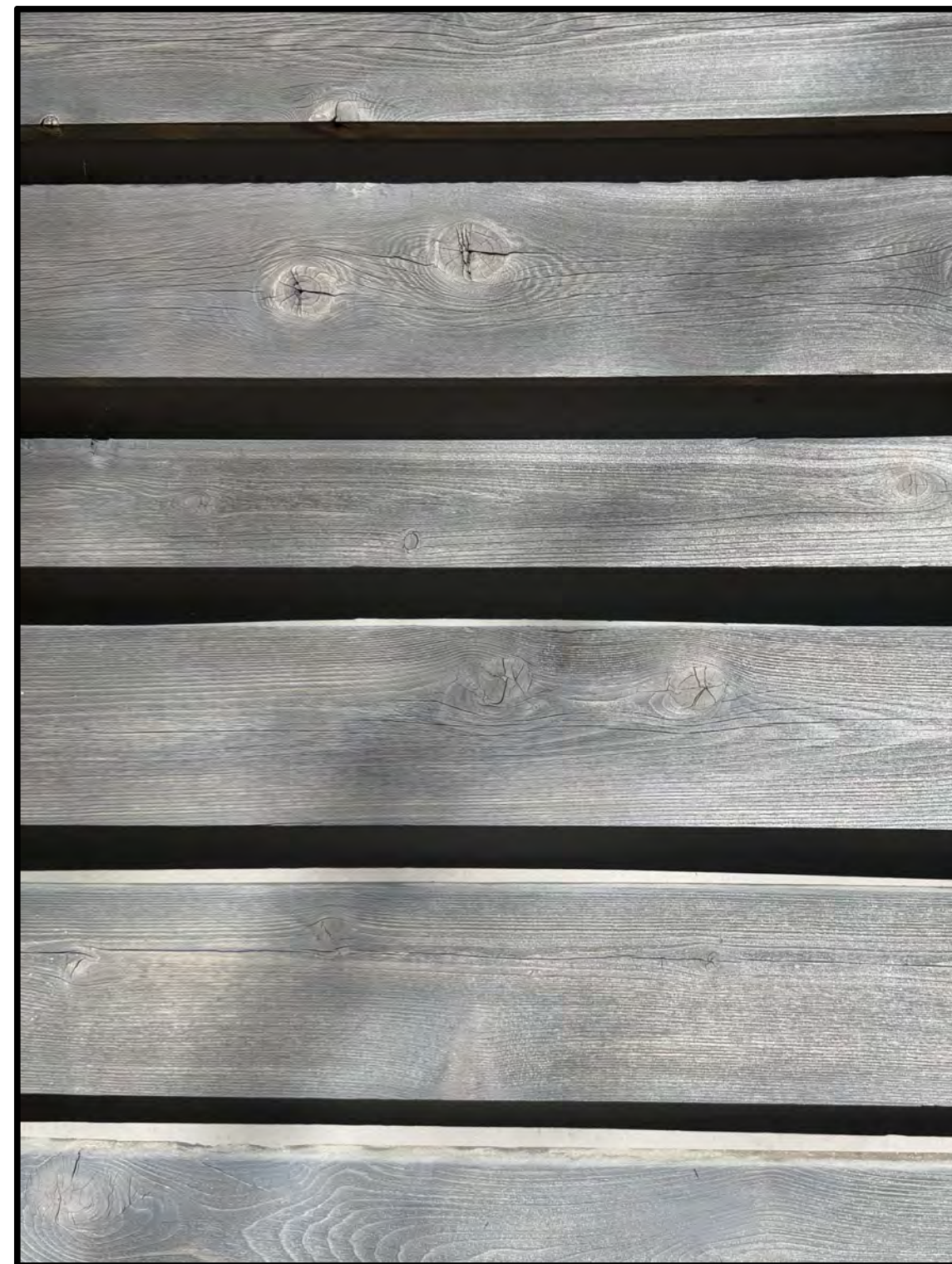
HORIZONTAL WOOD SIDING EXISTING EXTERIOR MATERIAL GRAY / BLUE STAINED CEDAR OPEN JOINT RAINSCREEN PROPOSED MATERIALS TO MATCH
