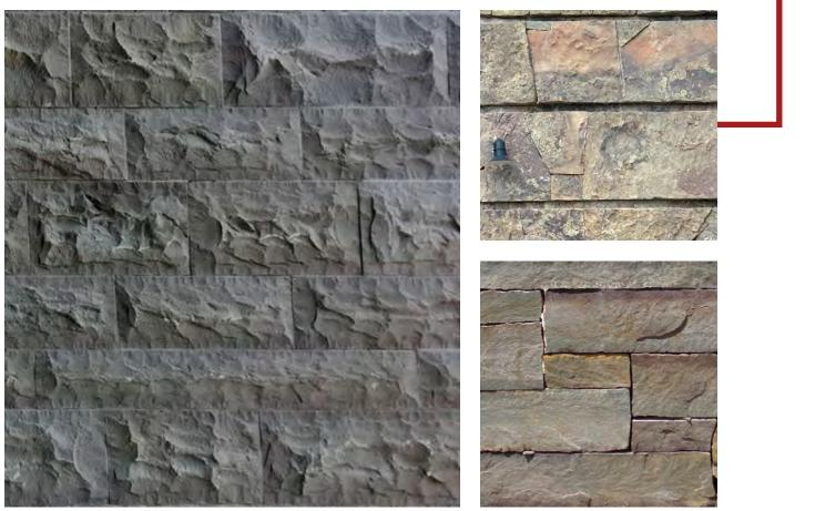
STONE VENEER - 4" thick natural stone with varying height. Dry-stack lay-up with stainless steel masonry anchor system.
