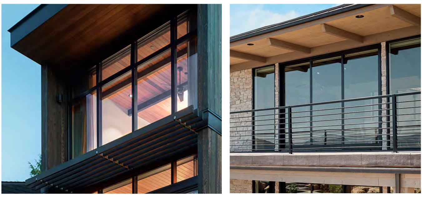
ALUMINUM WINDOWS AND DOORS - powder coated extruded aluminum with Low "E" insulated glass. Basis of Design: Vistaluxe Collection AL Line – Kolbe Windows and Doors. Basis of Design: Reynaers CP155LS Monorail System.
