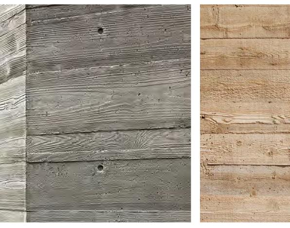
**BOARD-FORMED CONCRETE -** cast-in-place and stained.
