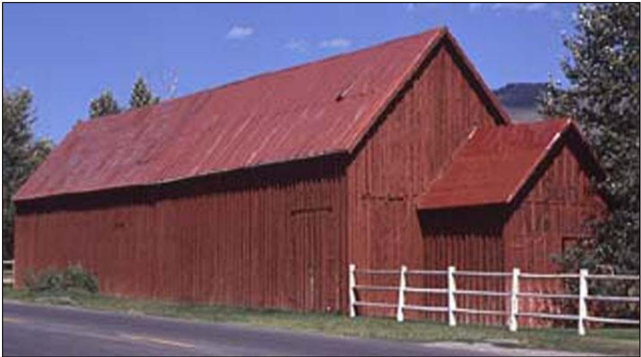
Figure 21. 1890 Lewis/Brass Barn on Sun Valley Road, view southeast.
