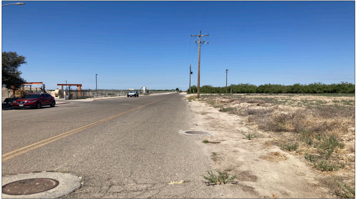
Figure 9. Photograph of a sewer line repair site, looking west from West Church Avenue, showing an inactive agriculture field and the wastewater treatment plant (left) with an orchard in the background.
