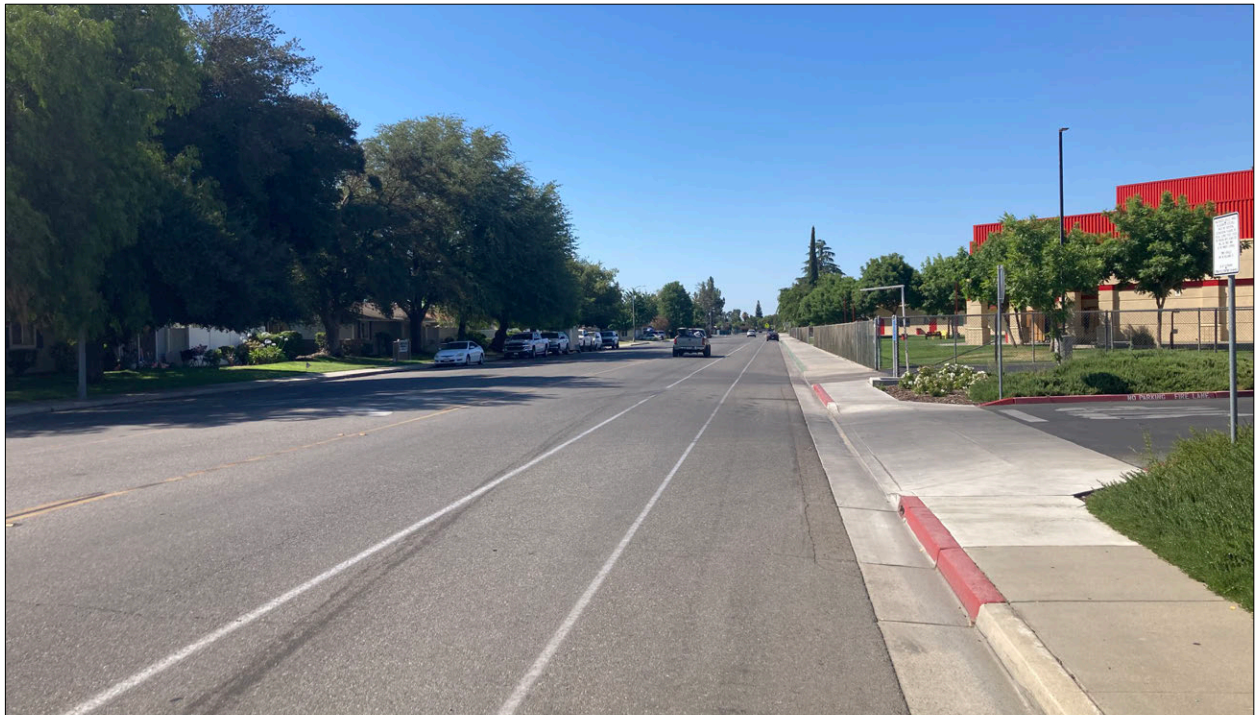
Figure 5. Photograph of a sewer line repair site, looking south along First Avenue, showing Kerman High School and residential development.
