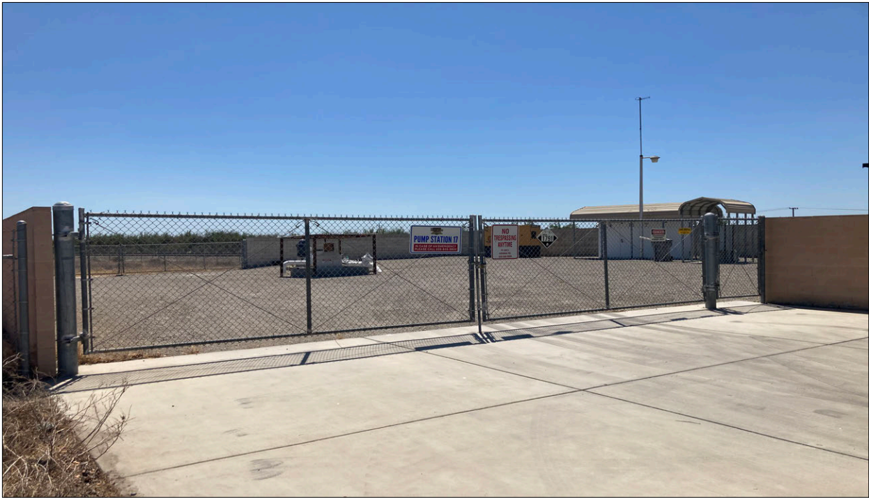
Figure 11. Photograph of the Lift Station Number 17 site, looking southeast from South Goldenrod Avenue.
