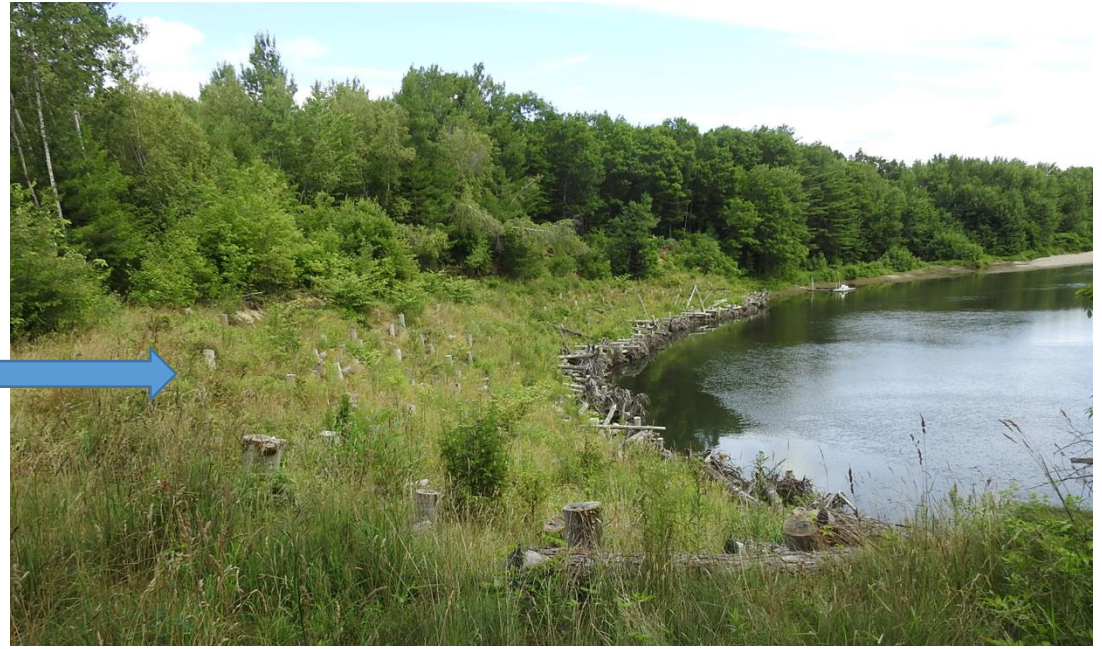
Near stream tree removal replaced with native plantings. Also shows bio-engineering to protect the toe.
