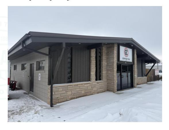
The applicant is requesting a variance to allow for the use of pro rib steel paneling for 10% of the façade. This paneling would wrap around the bottom half of the building and be the same height as the masonry. This is being requested for aesthetic reasons, and the applicant has stated he can remove it if necessary.
