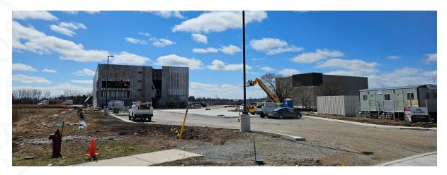
3. Legacy Creekside Apartments- The western most building has all the siding on and interior work is ongoing. One other apartment building is just starting to be framed up with the foundations in for two more apartment buildings.
