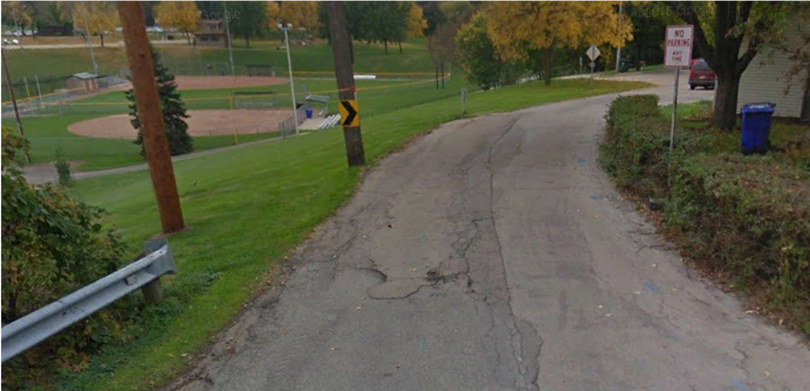
Tenth Street Looking Westerly from Alley
