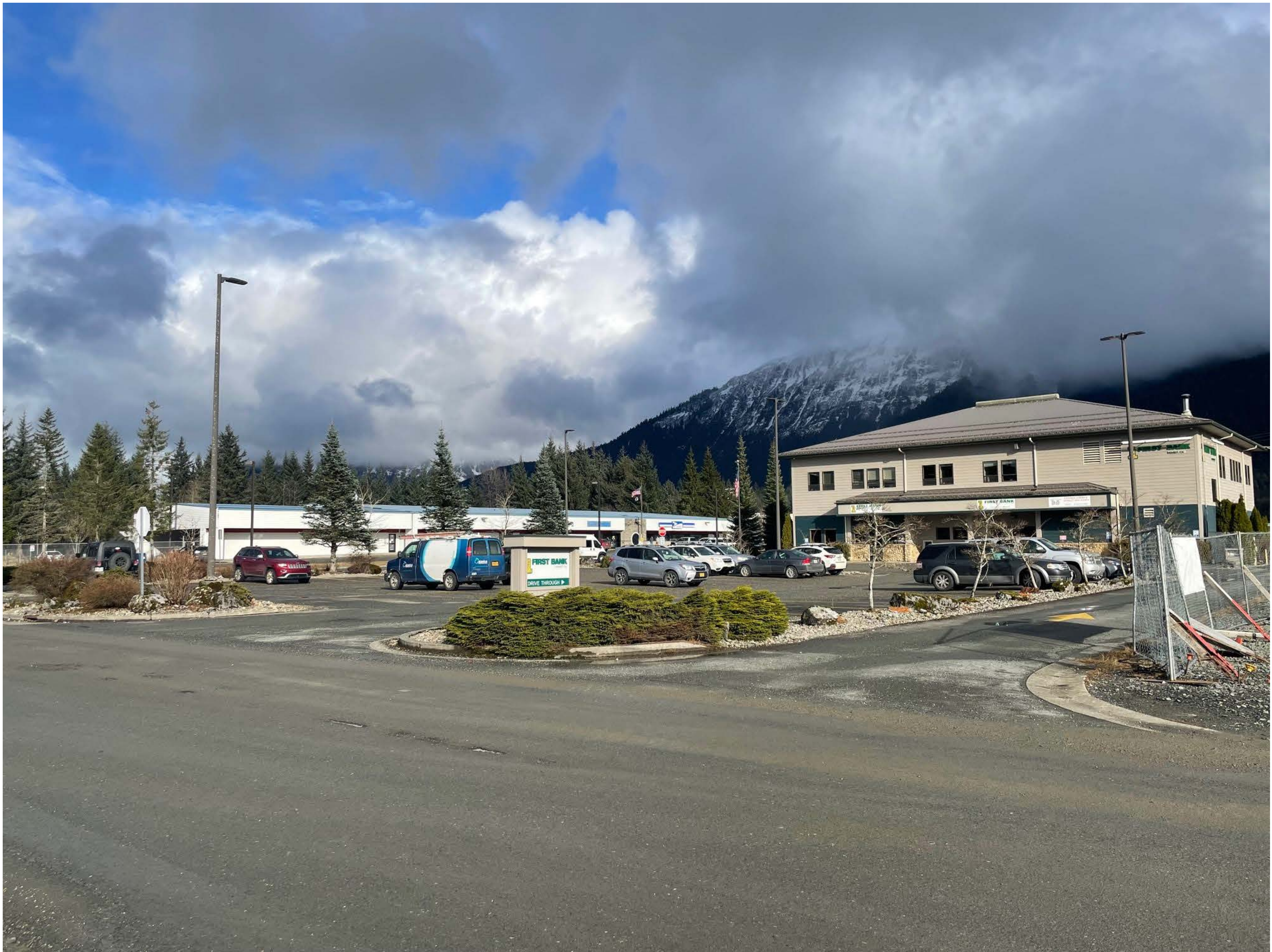
Attachment I - Site Photos
