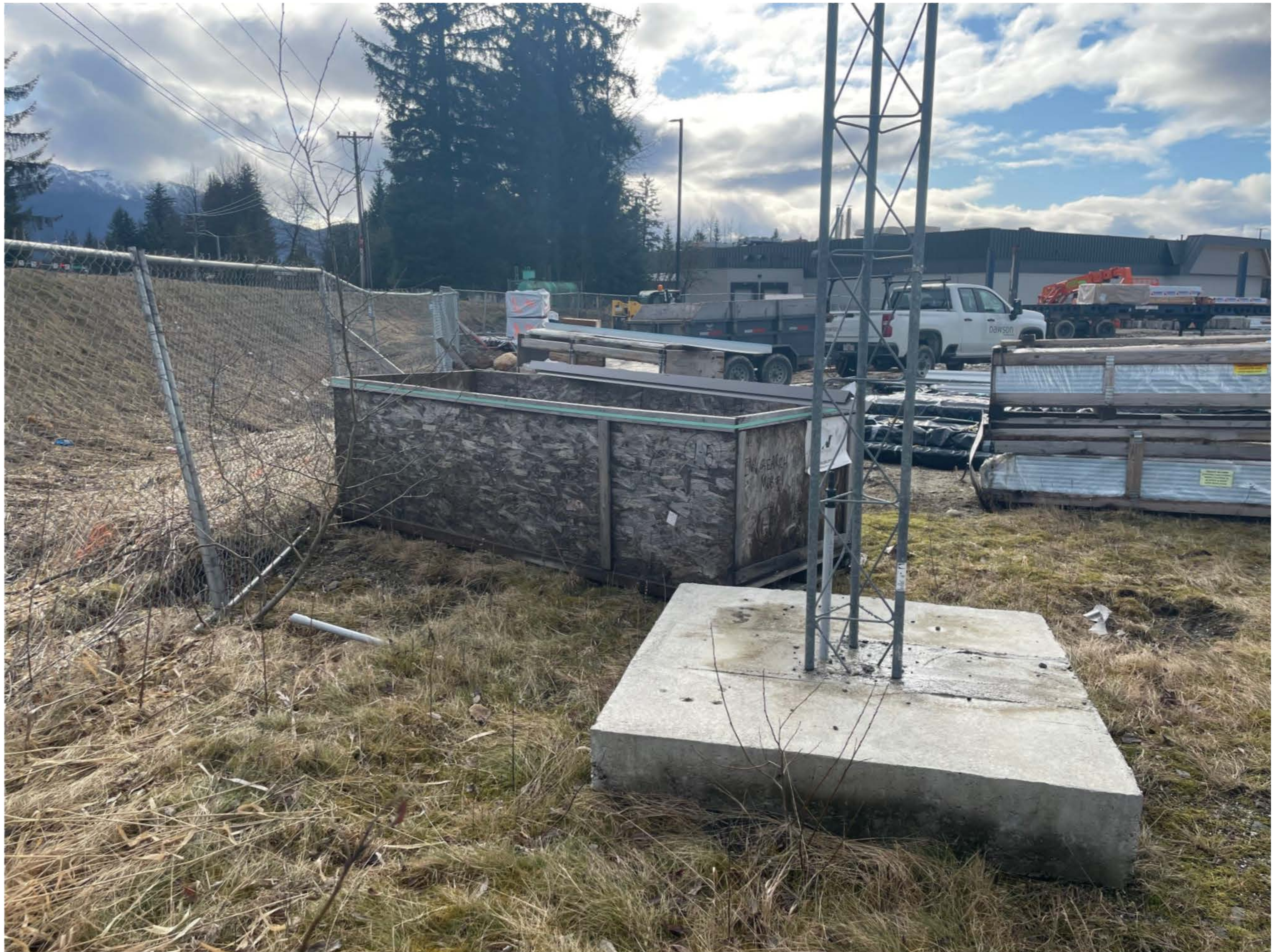
Attachment I - Site Photos
