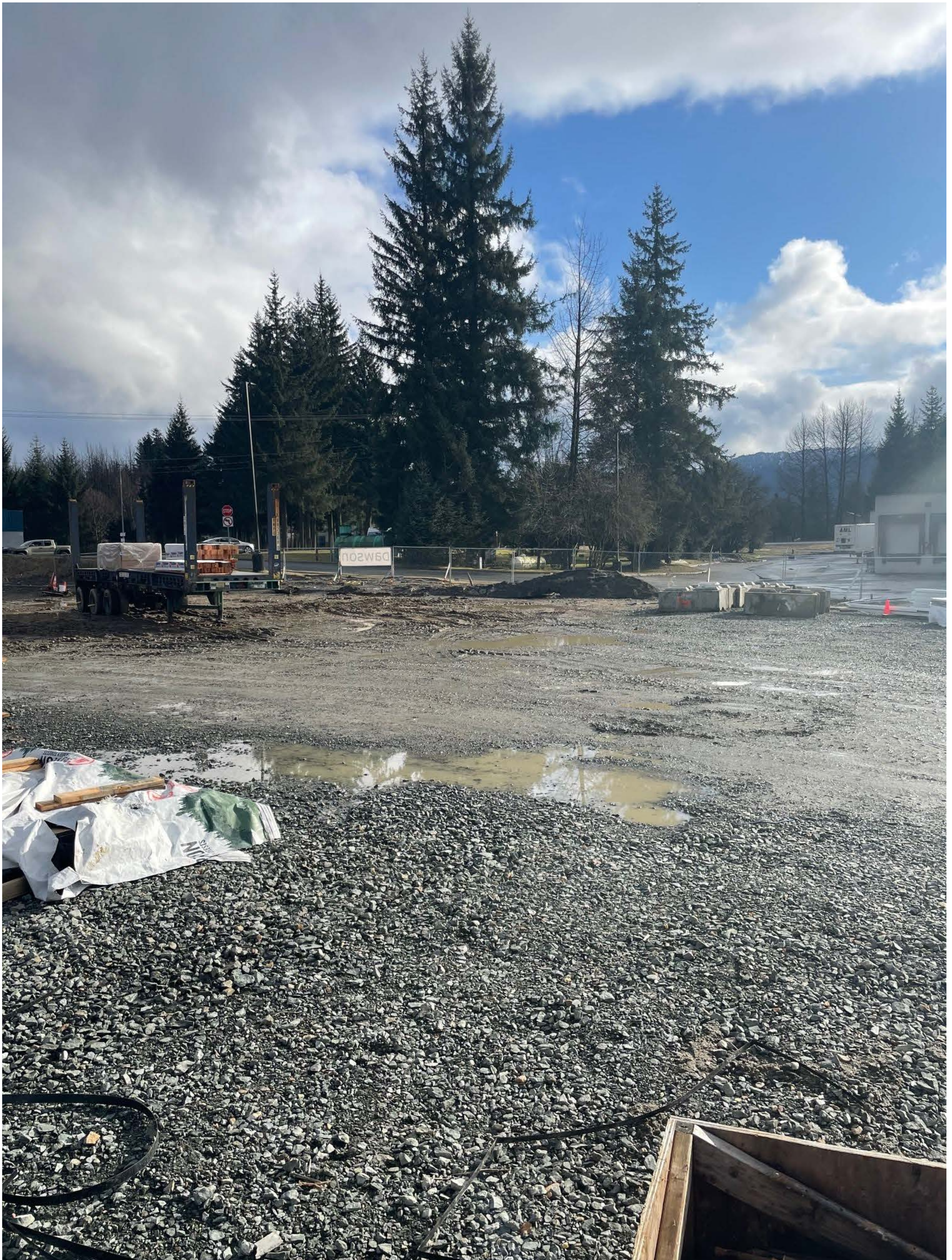
Attachment I - Site Photos
