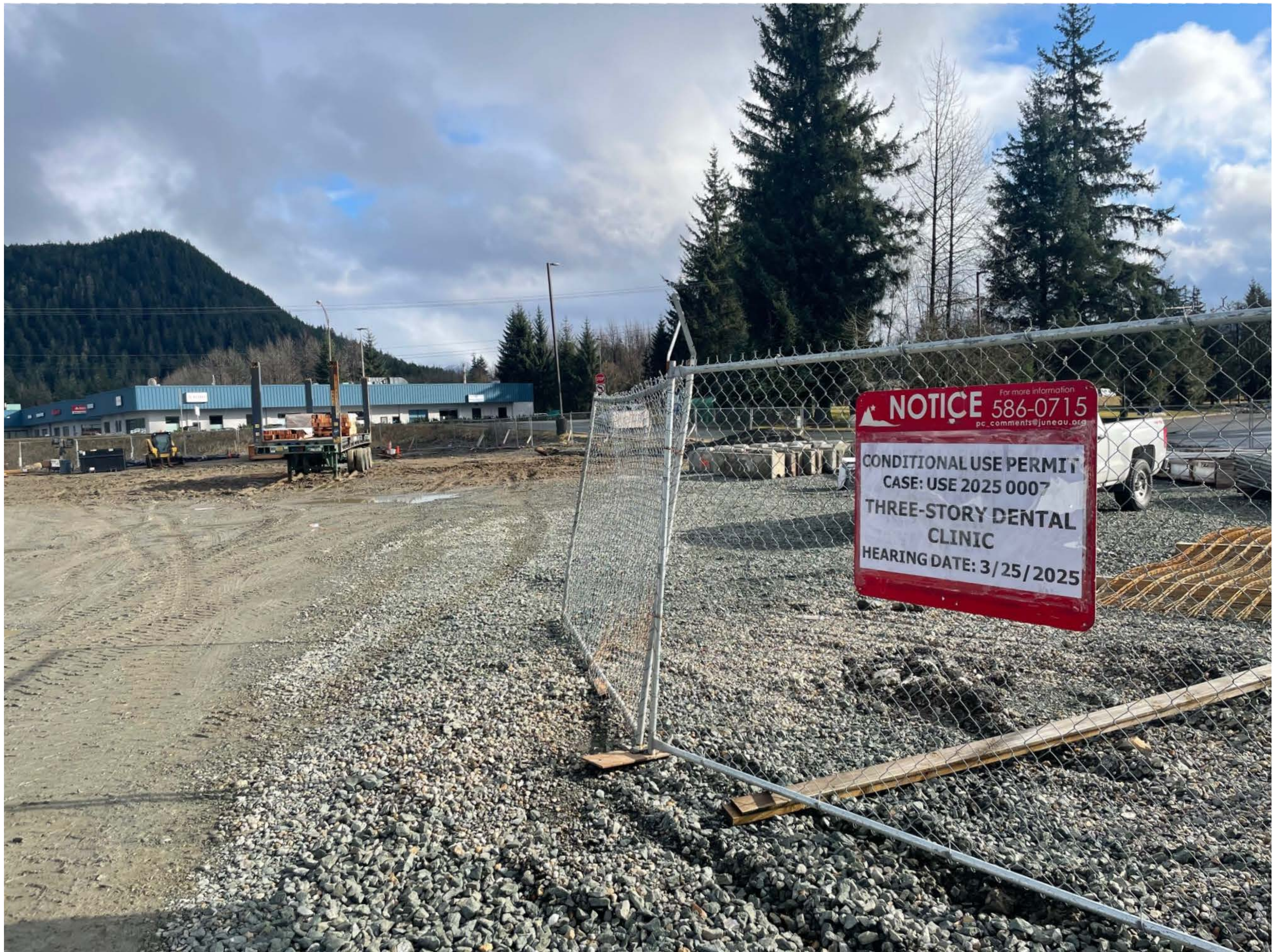
Attachment I - Site Photos
