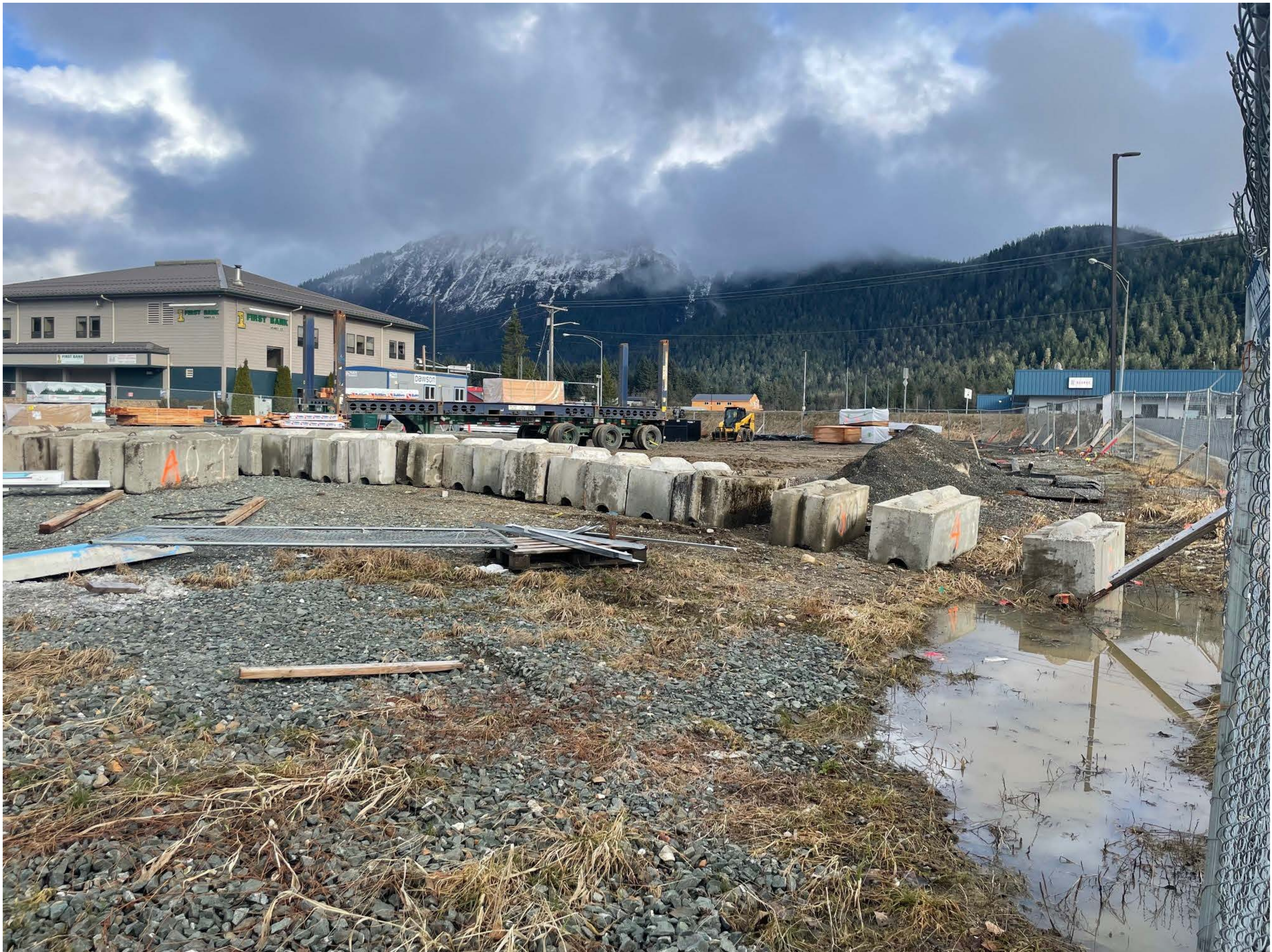
Attachment I - Site Photos
