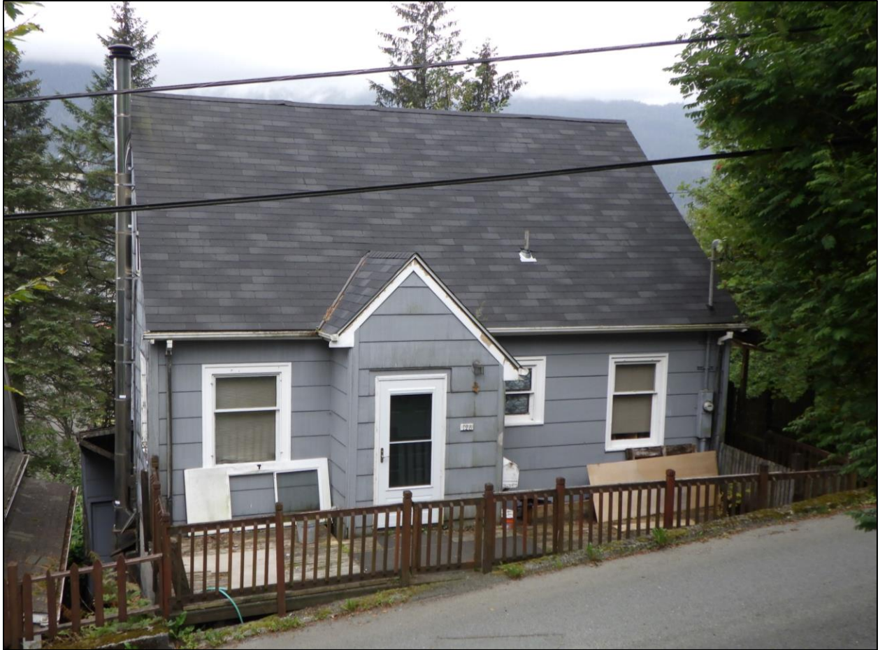
Figure 11. Looking west from Dixon St. at the Martin/Johnston House (JUN-00294) (NLURA photograph).
