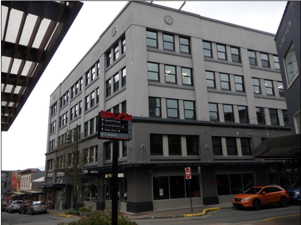
Figure 22. Looking Southwest at the Goldstein Building (JUN-00180) from the intersection of Seward and 2nd Sts. (NLURA photograph).
