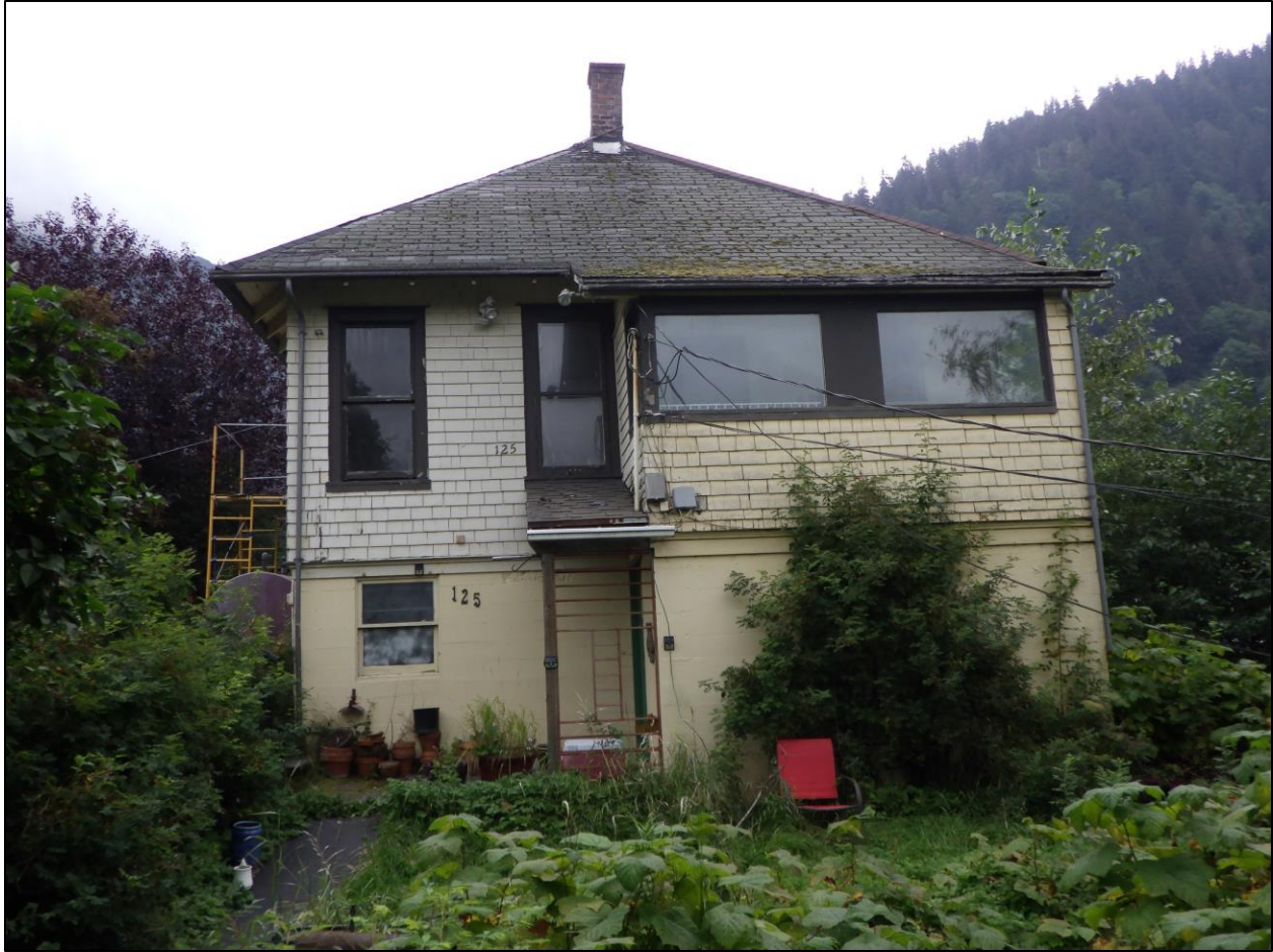
Figure 12. Looking east from Dixon St. at the Webster/Hurley House (JUN-00295) (NLURA photograph).
