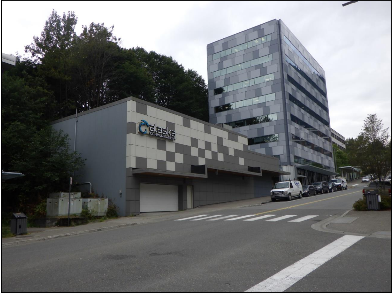
Figure 19. Looking roughly north west at the location of the Flag of All Nations Site (JUN-00080) (NLURA photograph). The AHRS point is in the center of Main St. .The Juneau and Douglas Telephone Company (JUN-01012) is the lower building in the foreground (NLURA photograph).
