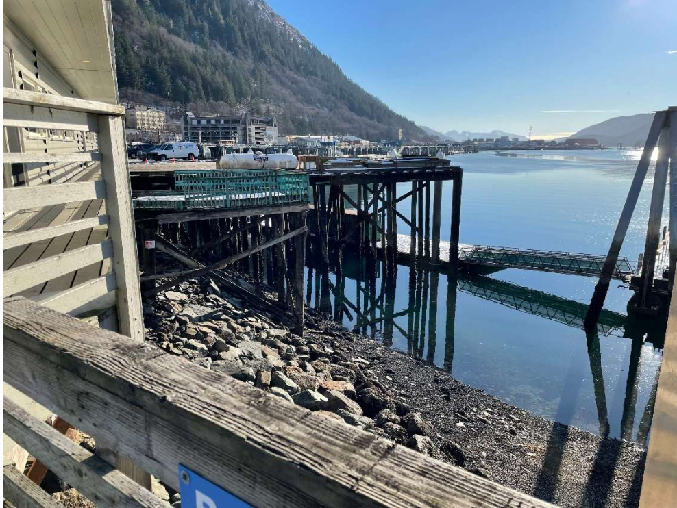
PHOTO 3 – View looking southwest across CX4.
