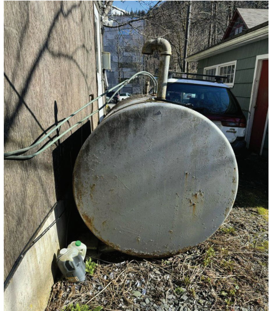
Fig. 20: Storage Tank at 203 West Third St.
