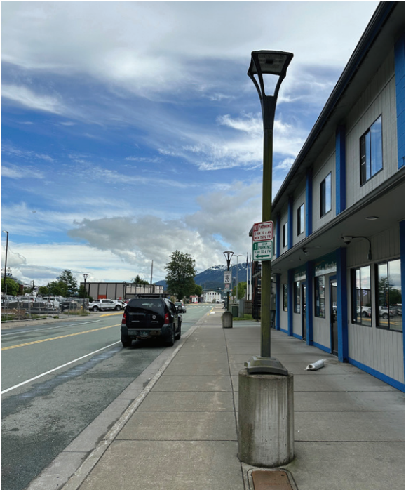
Fig. 43: Street Lighting Example
