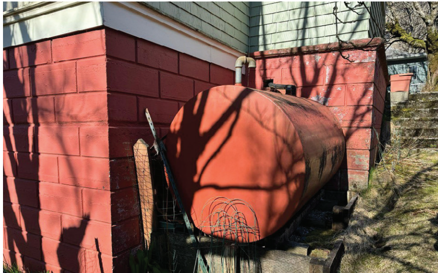
Fig. 19: Storage Tank at 214 Dixon St.
