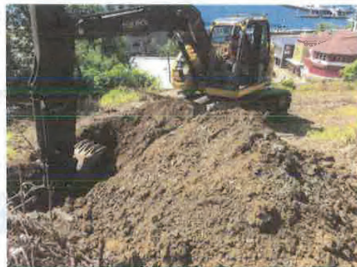
Figure 3: Excavator and in-situ silty sand with gravel
