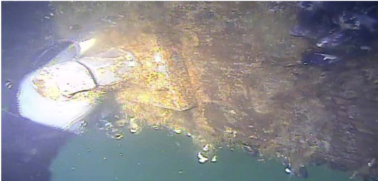
Figure 1 – Typical perimeter hardware, good condition and tight.
