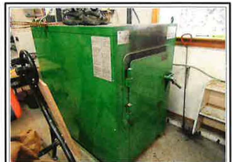
Wood and Oil Fired Boiler
