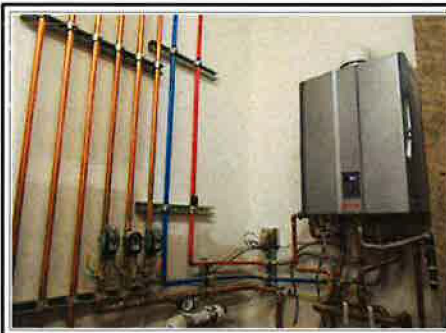
Boiler for the Accessory Unit
