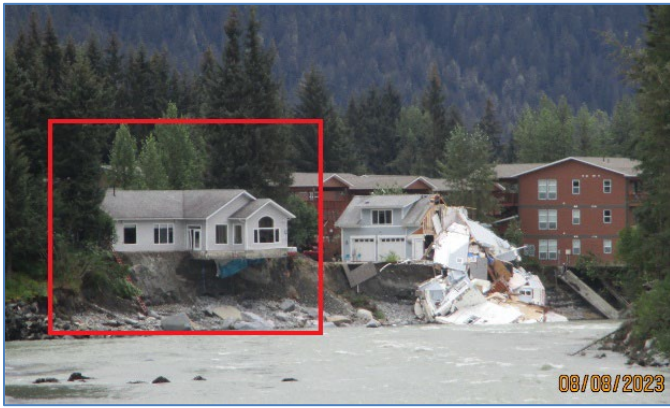
Washed out fill and cantilevered structure from flooding
