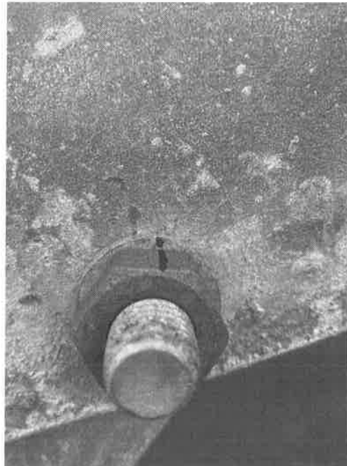
Photo 2 – (5/05/22) Mark of nut and washer for reference point for bolt tightening chart.
