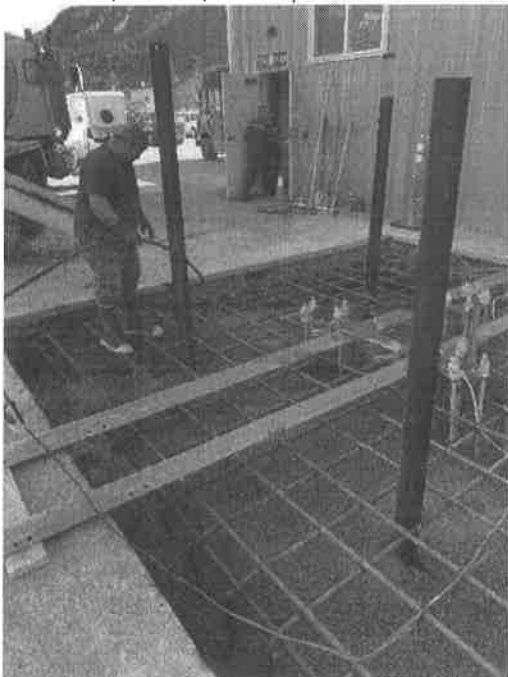
Photo 3 – (4/14/22) – Vibratory stinger being used to consolidate concrete.
