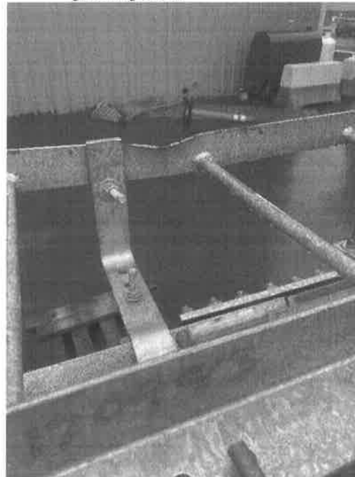
Photo 4 – (5/10/22) – Damage to one of the ladder sections.
