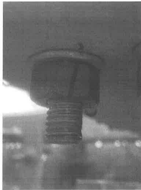
Photo 2 – (5/10/22) Mark of nut and washer for reference point for bolt tightening chart.
