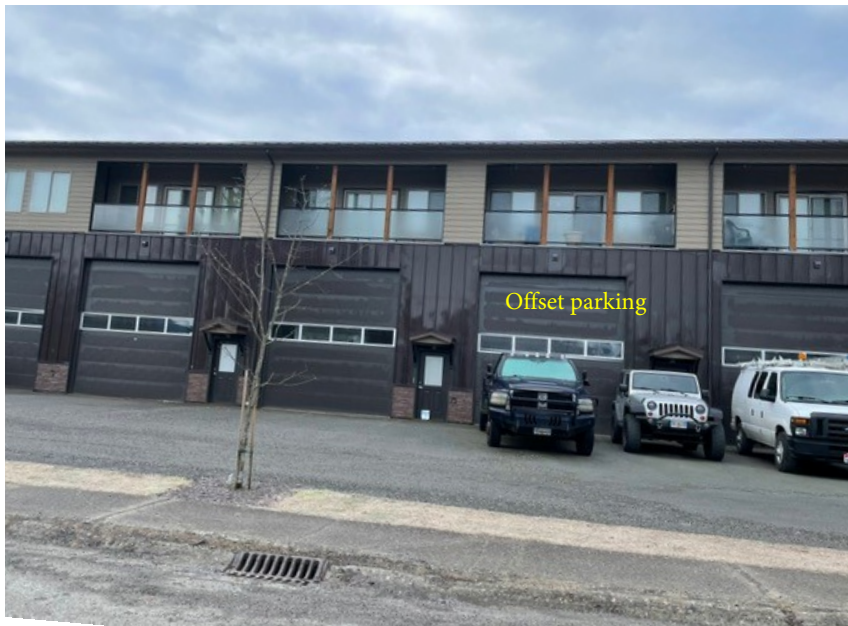
Attachment F - Site Photos
