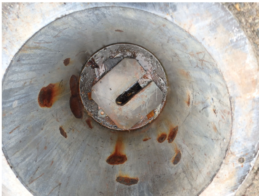
Photo 6. Inside of hawse pipe with chain keeper
