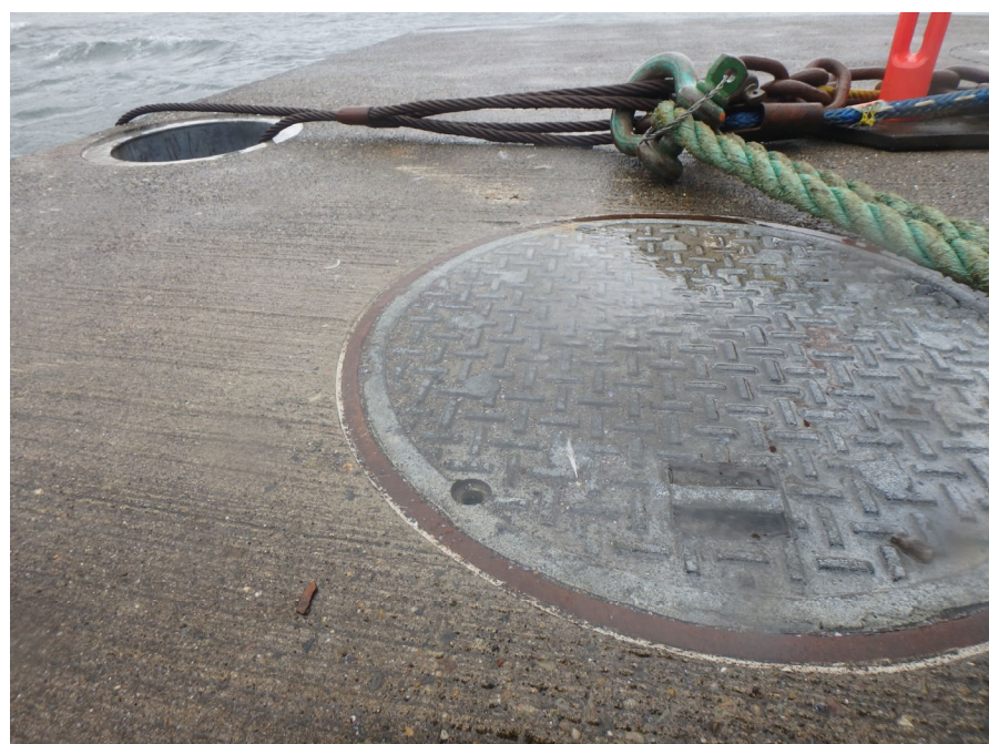
Photo 8. Hawse pipe and water tight manhole cover
