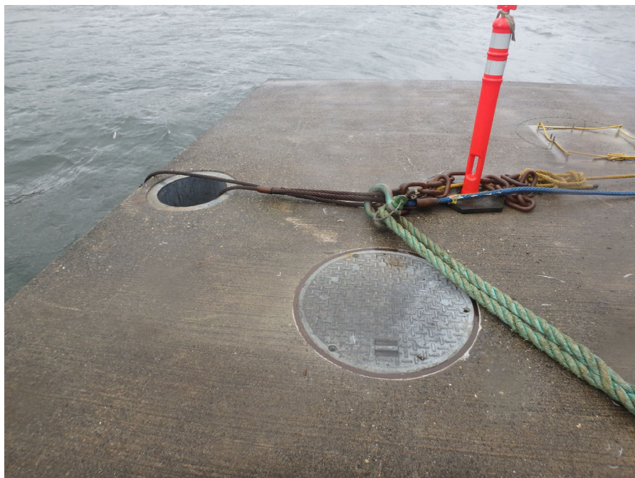
Photo 7. Hawse pipe and water tight manhole cover
