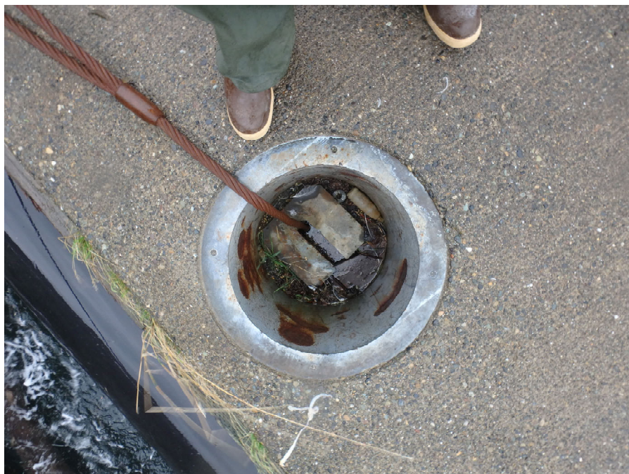
Photo 5. Inside of hawse pipe with chain keeper
