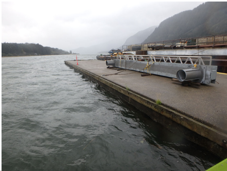
Photo 1. Overview of concrete breakwater float
