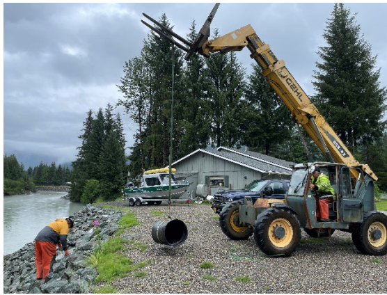
Figure 2 Image of installation of check valve at Rivercourt Way.
