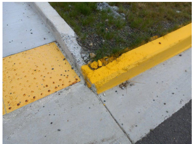
PHOTO 06: Damage at one of the accessible ramps.
