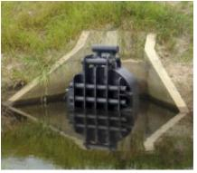
• In-line check valve: Is installed inside of the culvert with a pressure fit band sealing to the inside of the culvert. Functions similar to the duck bill – rubber diaphragm (intern to pipe) remains sealed except when inside water pressure is greater than the water pressure outside of the pipe. (outside water pressure is typically nonexistent except during flood events.)
