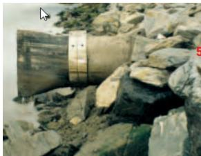
• <u>Flap Gate type:</u> hinged metal plate covering the end of the culvert outlet. Inside water pressure pushes the flapper open to drain the pipe. Outside water pressure pushes against the flapper to seal closed when the river water level is above the pipe outlet.
