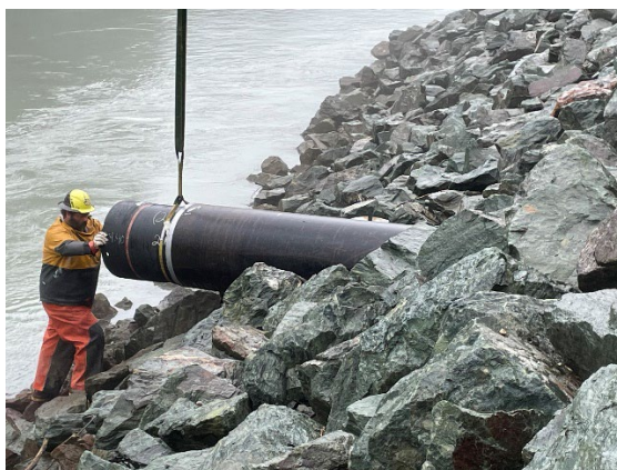
Figure 3 Image of installation of check valve at Rivercourt Way.
