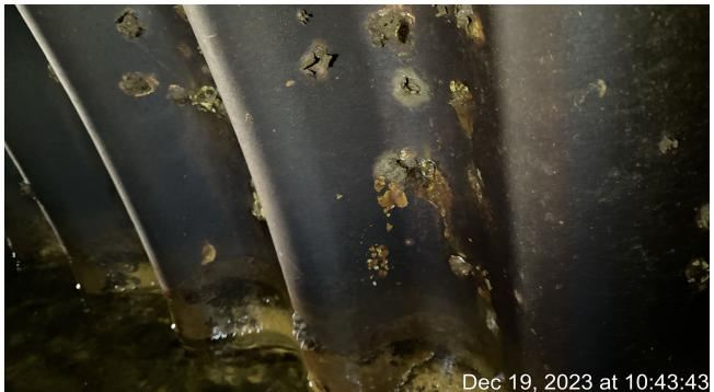
**Photo 01:** Heavy pitting and holes as observed on a portion of the half-arch culvert sidewalls. JNU staff has advised the FAA of the damage to this culvert, and of the very real possibility that it will need to be repaired or replaced. JNU has subsequently been advised that the work to repair or replace this culvert will **not** be AIP (Airport Improvement Project) eligible.
