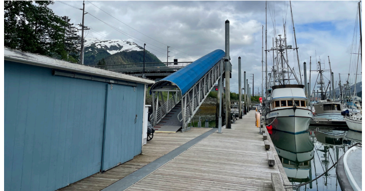
New head walk and gangway landing Float C installed as part of Phase I work.
