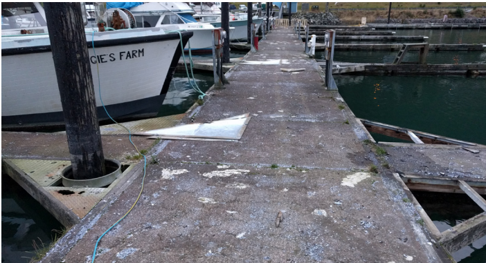
Deteriorated Phase IV floats prior to demolition.
