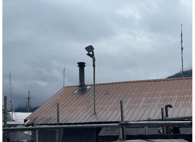
Aurora Harbor Outbuilding/Garage: Waste oil burner boiler stack has large amounts of mastic placed around perimeter to aid in reducing water infiltration.
