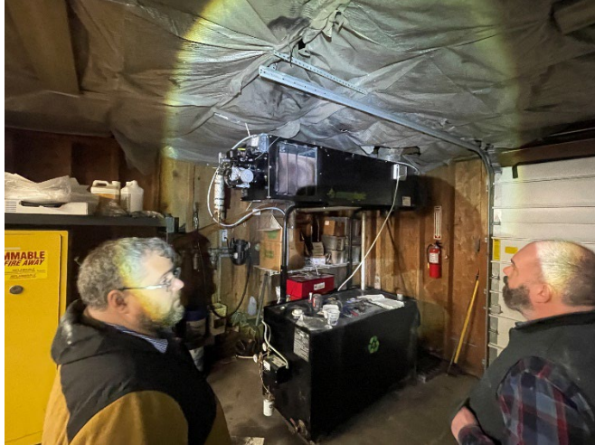
Aurora Harbor Outbuilding/Garage: View of waste oil burner in Garage area of Outbuilding.
