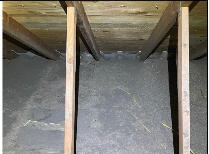
Aurora Harbor Office: Blown-in insulation should be tested for presence of ACM.
