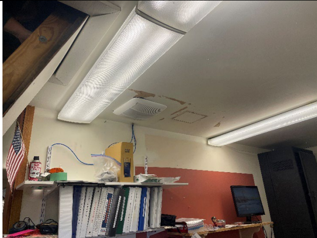
Aurora Harbor Office: Various fans in converted garage to Office area and main front office area have miscellaneous ceiling mounted exhaust fans that are piped into attic without proper roof or soffit vents.
