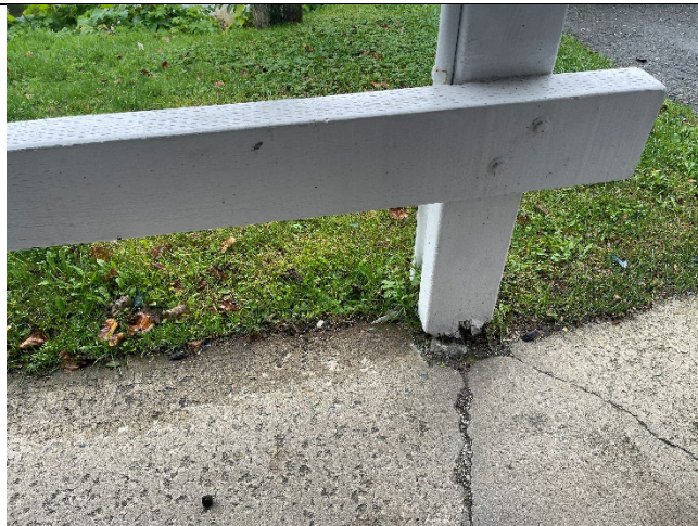
Aurora Harbor Office: Base of existing exterior canopy columns show signs of water damaged and are deteriorating.
