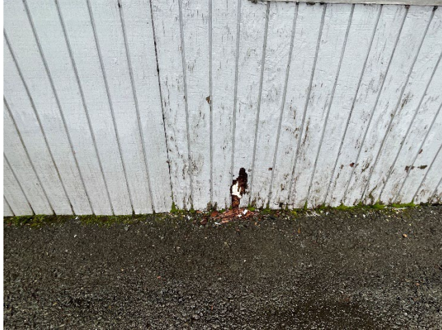
Aurora Harbor Office: Enlarged view of typical wood decay at siding.
