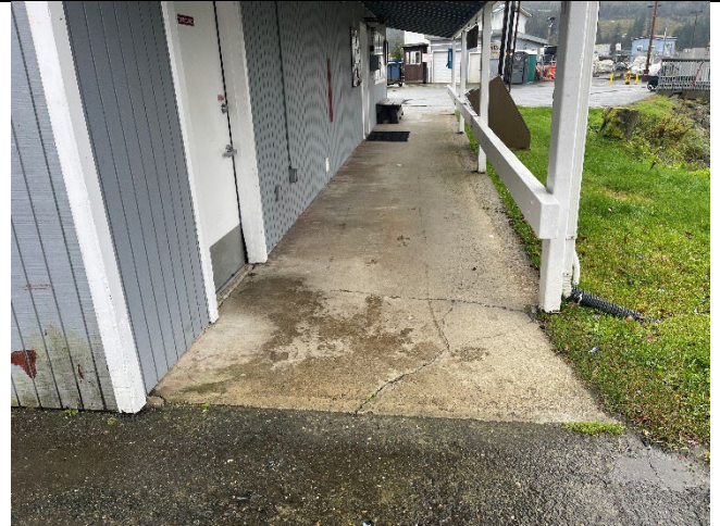
Aurora Harbor Office: Concrete sidewalk damaged and crackin along Northwest corner. Thresholds heights into office on the North end are not compliant with accessibility requirements.
