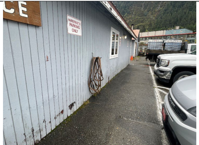
Aurora Harbor Office: Wood decay along base of siding. Appurtenances along face of structure sticking out into accessible isle.
