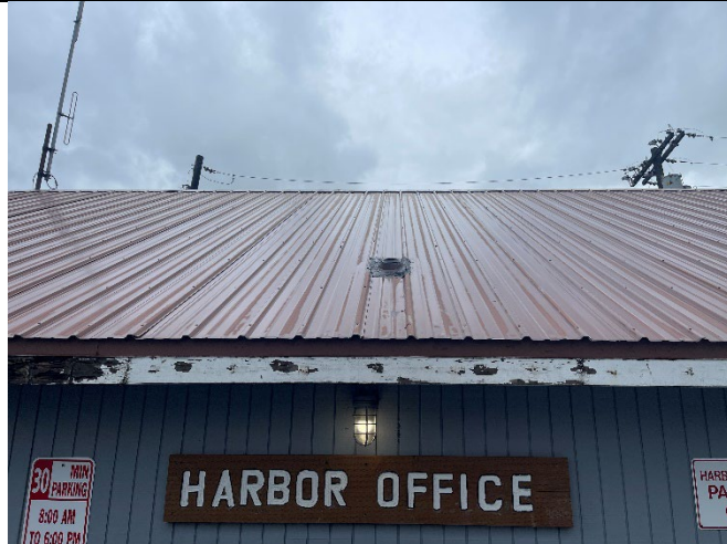
Aurora Harbor Office: Vent pipe between North and South bathrooms severed at roofline. General view of East side exterior water damage. Excessive wood decay present.
