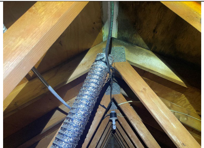
Aurora Harbor Office: View of misc exhaust fan not properly vented.
