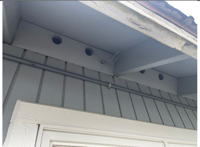
Aurora Harbor Office: Various abandoned wiring present around building outside of j-boxes.
