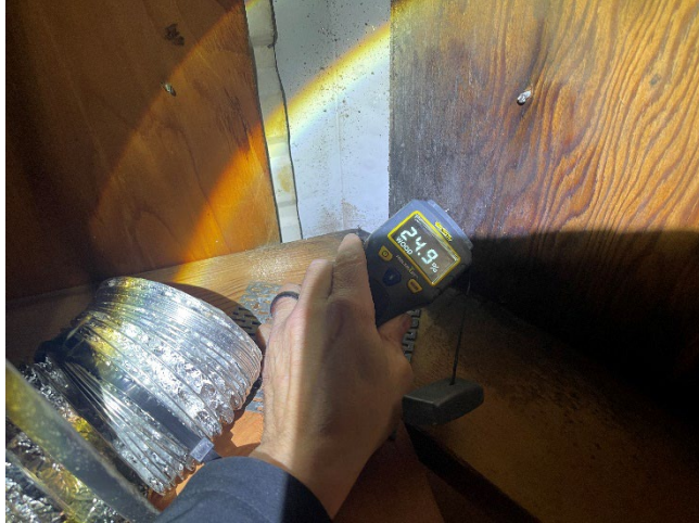
Aurora Harbor Office: View of misc exhaust fan not properly vented. High moisture content in plywood sheathing and mold present on deck and framing.
