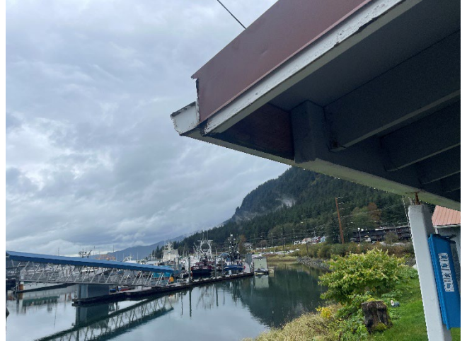
Aurora Harbor Office: Wood decay present at eaves where gutters remain intact.
