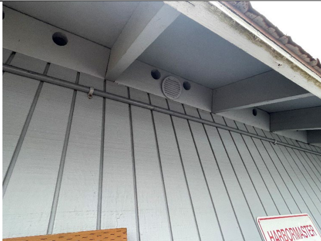
Aurora Harbor Office: Bathroom vents with non-compliant vent louvers, typical.
