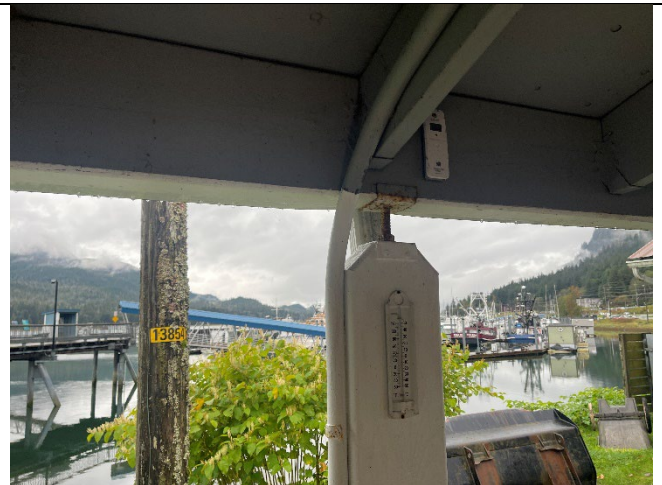
Aurora Harbor Office: Tops of columns do not appear to be appopriate use of the type of post bracket. The use of an adjustable bracket also relays that its use may be due to structural movement of the columns that should be addressed.
