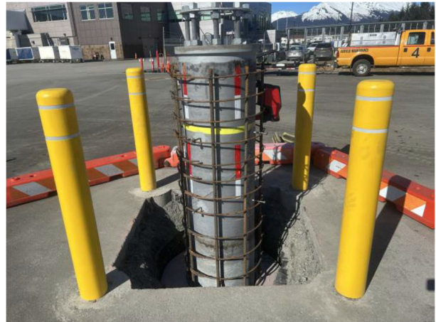
PHOTO 02: Typical Reinforcing Installed Around the Piling
