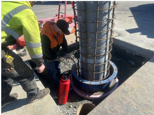
PHOTO 03: Form Base Set in Position at LP-5
