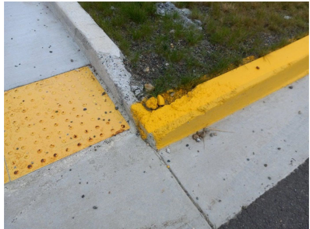
PHOTO 06: Damage at one of the accessible ramps.
