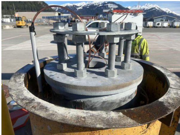
PHOTO 01: Typical Pile Cap Assembly
