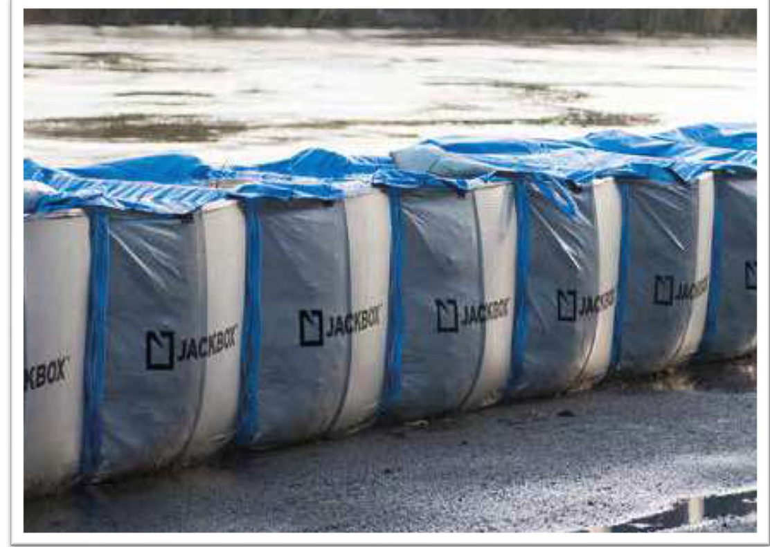
HESCO Barriers Installed Along a Riverfront
