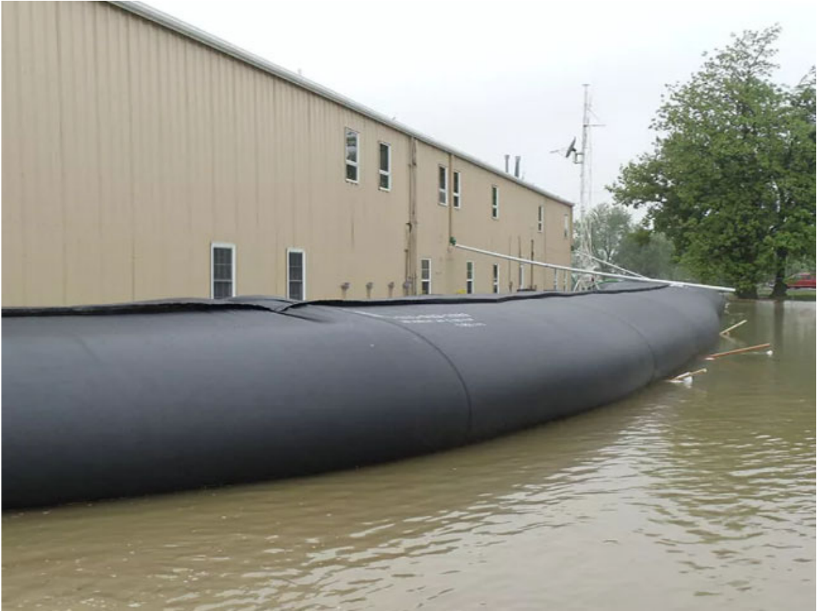
Water Filled Sandbag Equivalent Levee
