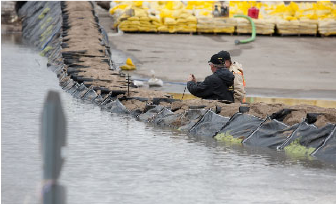
Sand filled Levee System
