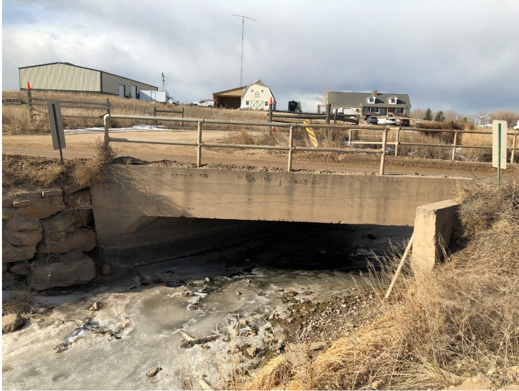
Figure 3 - Existing Structure at Hillsboro Ditch
