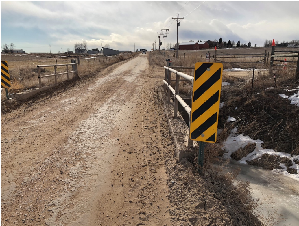
Figure 4 - Existing Roadway at Hillsboro Ditch
