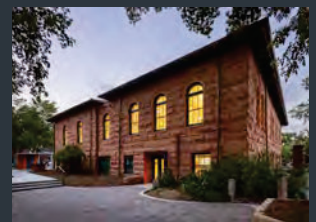
Before and after of the exterior. During demolition, the project team carefully removed the original windows and sent the windows offsite. The glass was restored and reused in the finished project.
