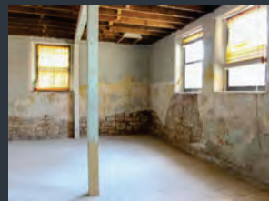
Before and after of the first-floor meeting room. During the renovation, the project team decided to leave portions of the wall exposed to the underlying, original sandstone brick.
