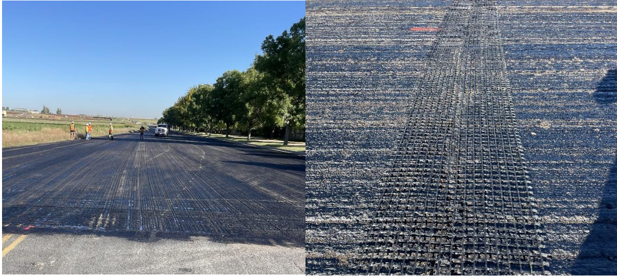
Colorado Boulevard Overlay
