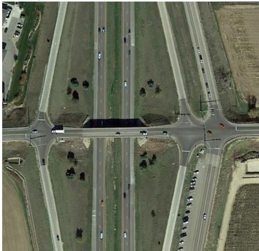
Figure 2. Current Condition of SH 60 Interchange
