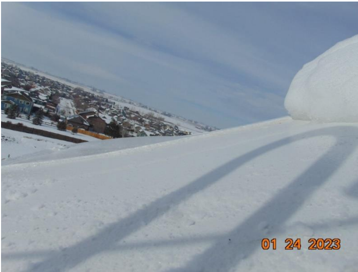
Exterior Coating / Roof
