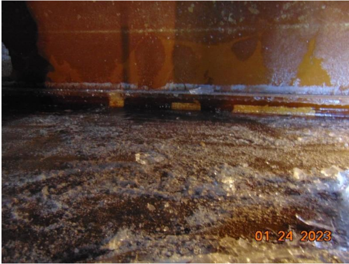
Floor / Shell Connection
