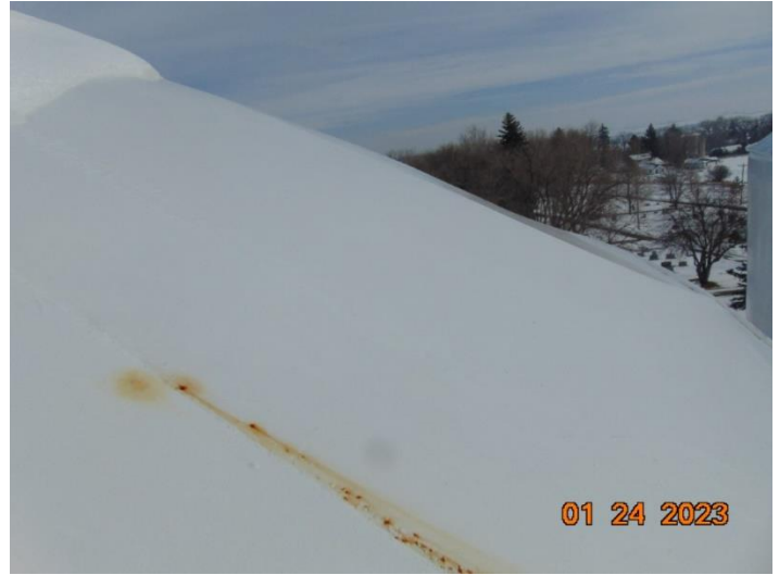
Exterior Coating / Roof
