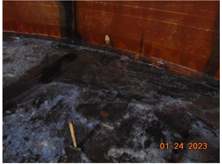
Floor / Shell Connection
