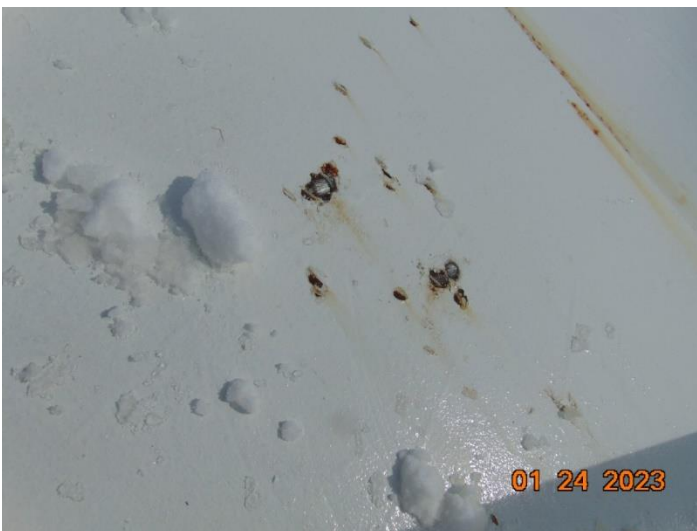
Exterior Coating / Roof
