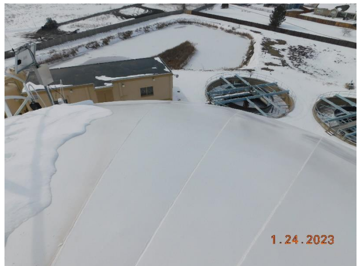
Exterior Coating / Roof
