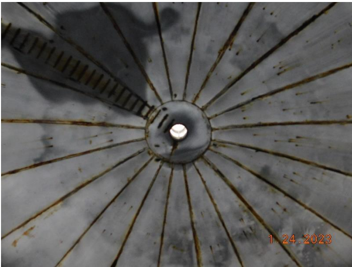
Roof Interior from Floor
