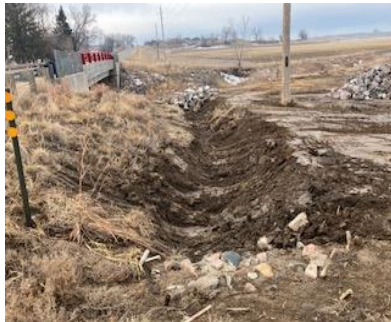
Rip Rap Installed on WCR 17 at Little Thompson River for Bridge Stabilization and Erosion Control
