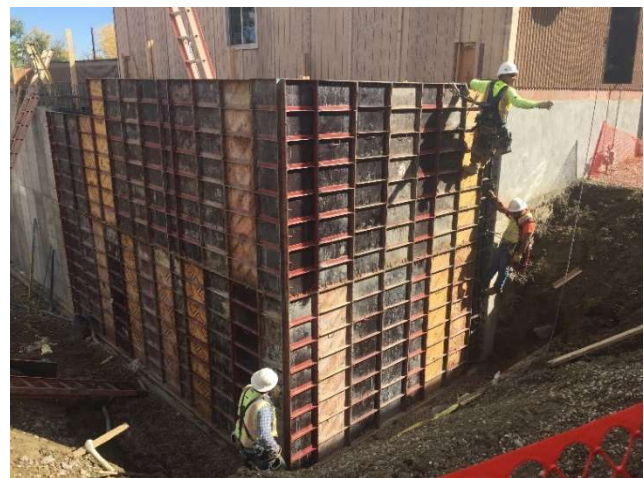
Photo: Construction of the New Filter Trains #3 and #4
