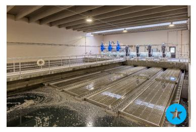
Burns & McDonnell worked as part of a design-build team with Garney Construction to upgrade to the Dodd Water Treatment Plant (DWTP) in Niwot, Colorado. Burns & McDonnell permitted and designed and the upgrades to the DWTP. The DWTP includes conventional pretreatment with high-rate inclined plate settlers, MF/UF membranes, clearwell, and high service pumping to increase capacity from an 8 MGD to 10 MGD with the capability to expand to 16 MGD.
