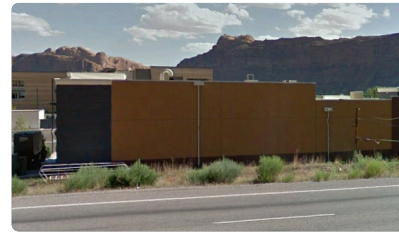
Colorado River Resort WTP
