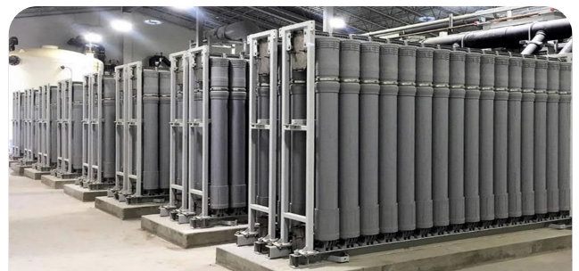
Pressure membrane modules provide a compact footprint in comparison with conventional media filters.
