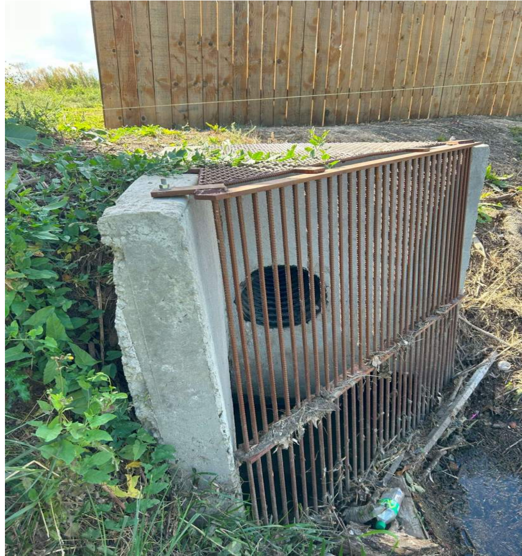
Existing Pond Outlet
