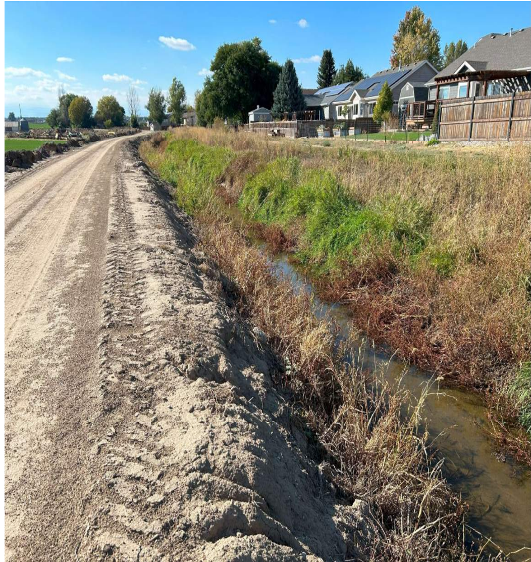
Hillsborough Ditch Looking Downstream
