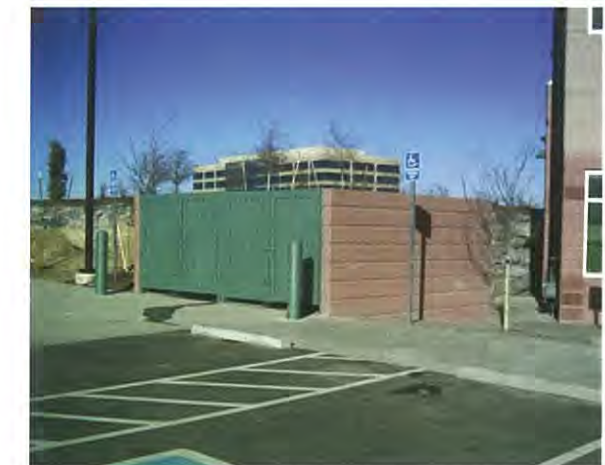
EXAMPLE OF TRASH ENCLOSURE WITH BOLLARD PROTECTION.
