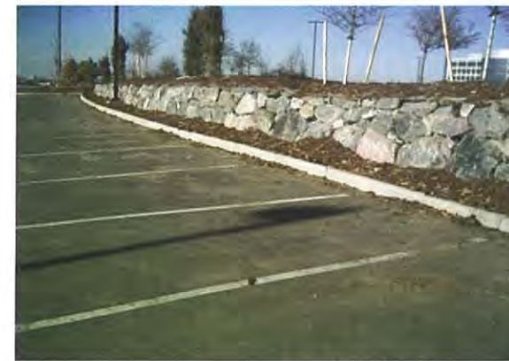
EXAMPLE OF STONE RETAINING WALL.
