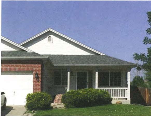
EXAMPLE OF HOME WITH COVERED FRONT PORCH
