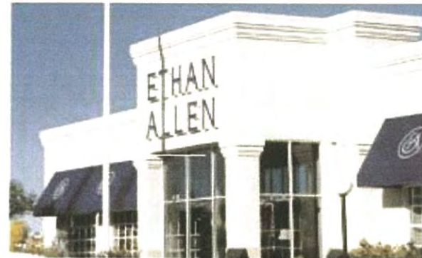
EXAMPLE OF ONE STORY BUILDING WITH STUCCO AND AWNINGS
