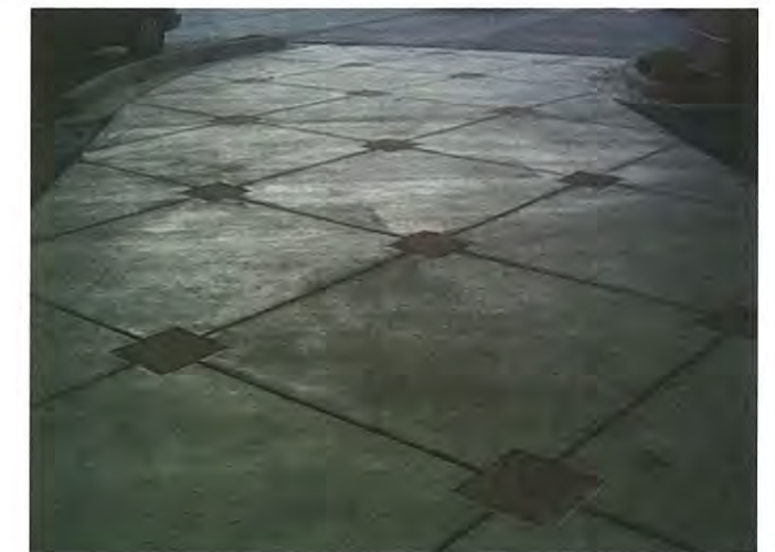
USE BRICK PAVERS, RECESSED STONE AND COLORED CONCRETE IN PEDISTRIAN ROUTES AND DROP OFF AREAS.
