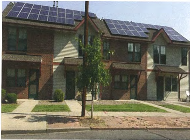
EXAMPLE OF TOWNHOMES WITH SOLAR
