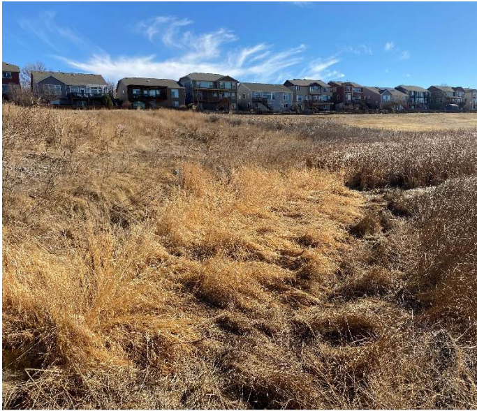
Stormwater Conveyance Channel
