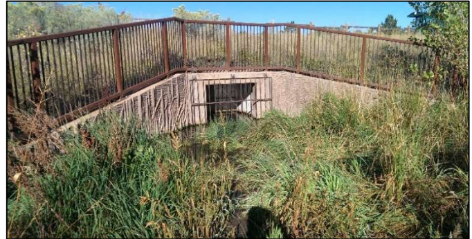
Outlet Headwall with Form Liner
