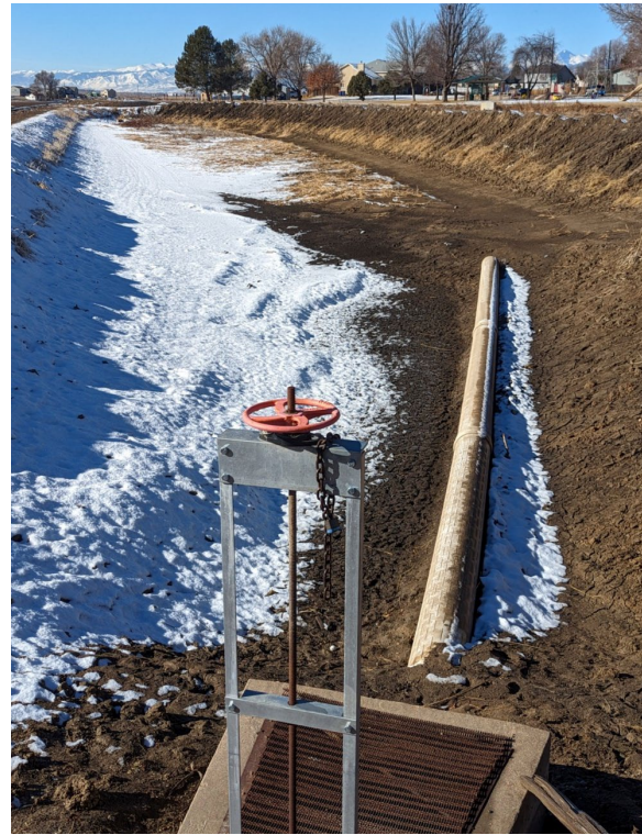
Possibly a relief basin adjacent to Hillsboro Ditch
