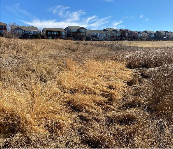
Stormwater Conveyance Channel
