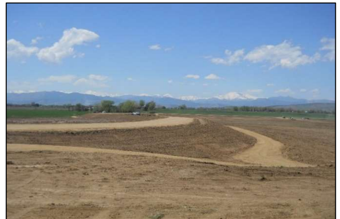
Completed Embankment for the TLN Regional Detention Pond (Prior to Revegetation)
