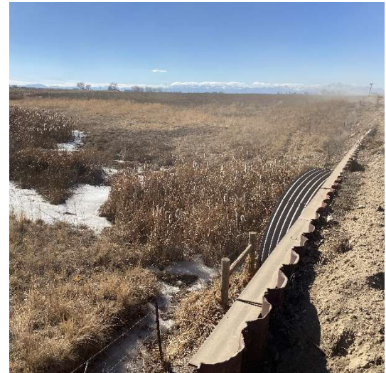
Bunyan Basin Crossing of County Road 42
