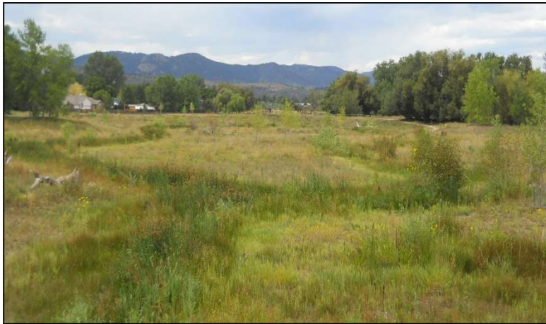
Completed Red Fox Meadow Detention/Water Quality Pond
