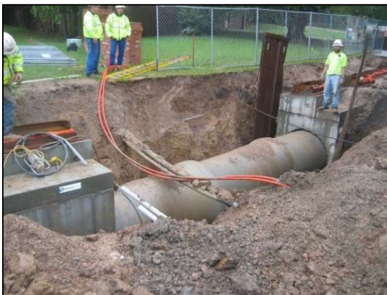
Storm Sewer and Inlet Installation on Suffolk Street
