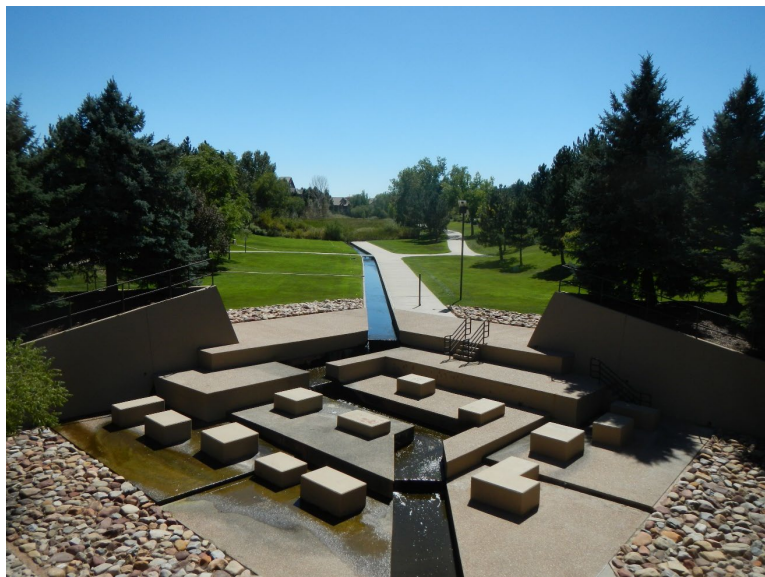
Goldsmith Gulch drop structure.
