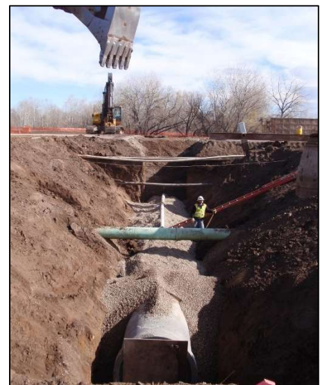
Storm Sewer Crossing at Taft Hill Road
