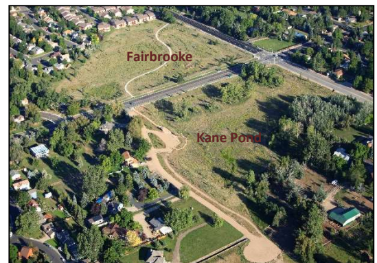
Completed Detention Ponds – Fairbrooke and Kane
