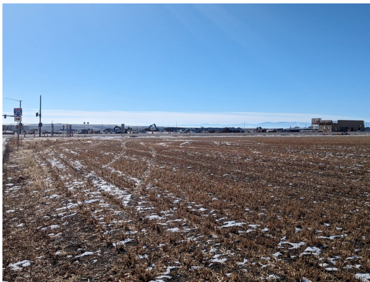
Agricultural Fields and Construction Project near I-25
