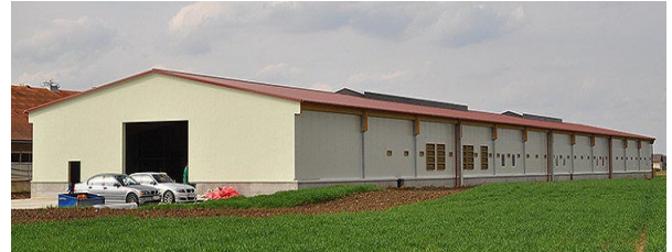
Figure 2-34 Unacceptable Metal Panel
