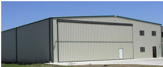
Figure 2-39 Unacceptable Metal Panel
