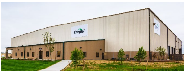
Figure 2-37 Unacceptable Metal Panel
