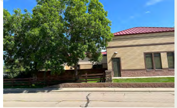
MWGC will assess all elements for the new additions and renovations.
