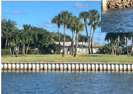
Photos at low tide, show +2-3 feet capacity
