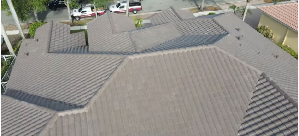
Picture of the Espresso Blend Roof tile installed
