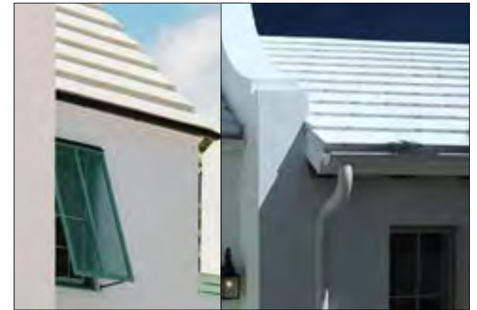
CLAY TILE IS USED MOST FREQUENTLY FOR ROOFING MATERIAL
