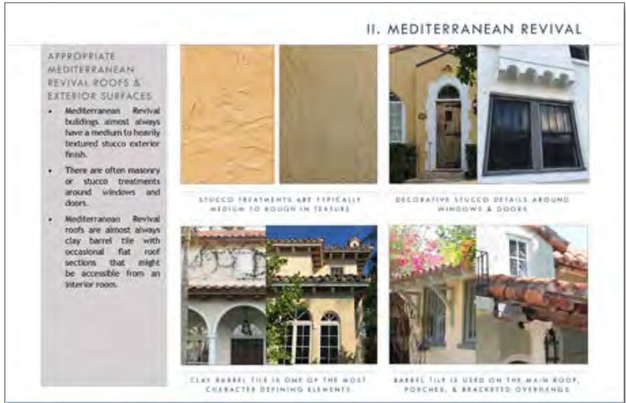
Excerpt of from the sample Architectural Design Guidelines found in Appendix D.
