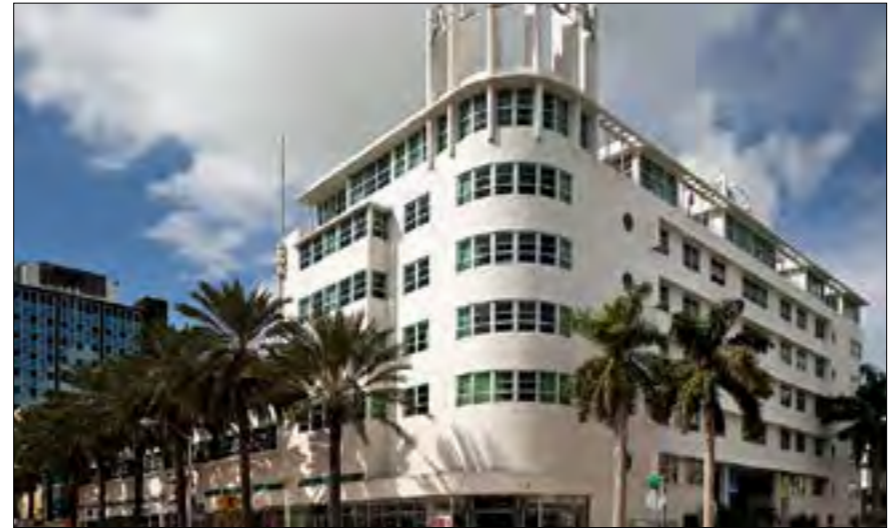
Figure 50 Albion Hotel, Miami Beach, FL
