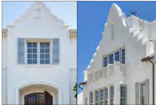
SCULPTED CONCRETE PARAPET WALLS ARE A CHARACTER DEFINING ELEMENT
