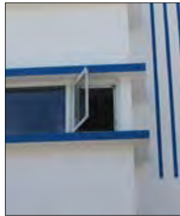
FIXED-PANE GLASS WITH SINGLE PANE CASEMENT
