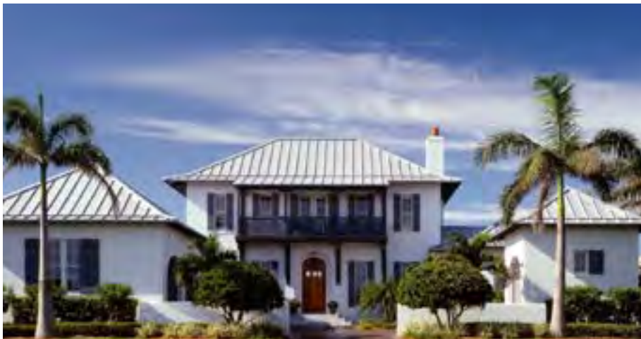
Figure 34 Purdum Residence, Tampa, FL, Cooper Johnson Smith Peterson Architects & Town Planners
