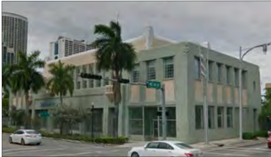
Figure 48 Office Building, Miami, FL
