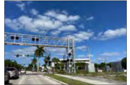
View of the FEC railway crossing at Tequesta Drive (looking West).
