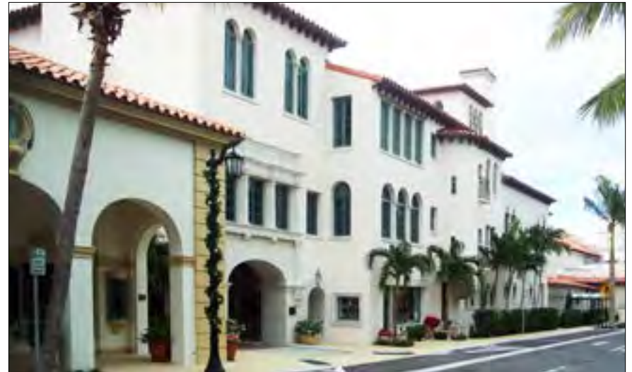
Figure 40 Everglades Club, Palm Beach, FL Architect: Addison Mizner.
