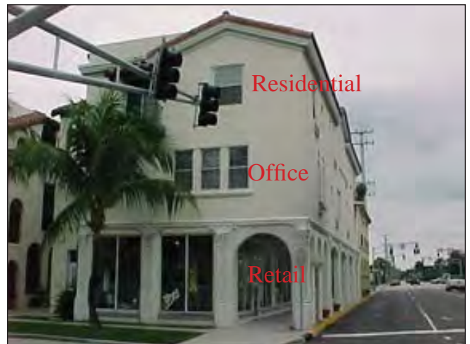
Mixed use building integrating retail office and residential uses in Palm Beach, Florida.
