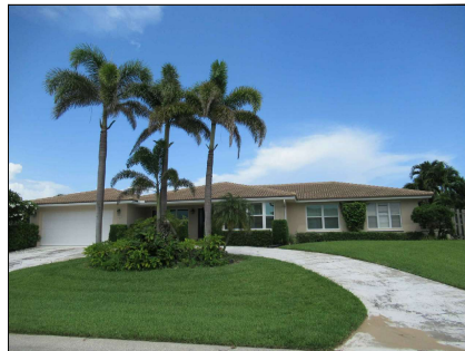
530 N LYRA CIRCLE (2ND RESIDENCE ACROSS STREET, EAST SIDE)
