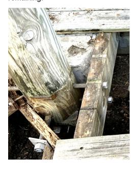
The wood column of the gazebo appears to be good despite some deterioration of the adjacent wood framing.
