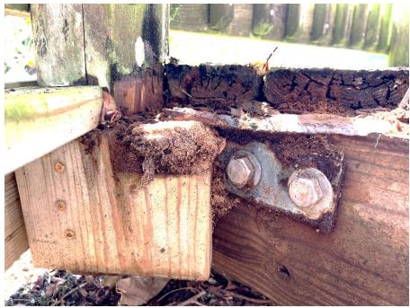
This enlarged photo shows the angled floor joist at a connection located at the octagon-shaped railing post. The framing and steel connections are complex and unusual in their configuration. The stainless-steel bolts are in contact with dissimilar carbon steel connector plates which has succumbed to galvanic corrosion. Some of the odd sizes and shapes of wood appears to have been constructed with wood that was not preservative treated lumber.
