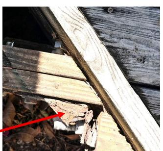
Many of the odd sizes and shapes of wood members in the extended deck exterior to the gazebo columns and interior octagon deck appear to have been constructed with wood that was not preservative treated lumber. The perimeter wood framing, decking and connections are generally in poor condition. (See left and below)
