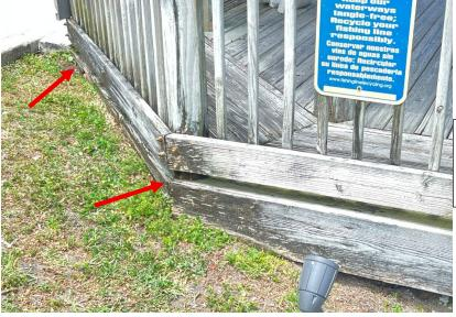
Note that this wood near the soil and sidewalk is more distressed than wood with air circulation. (South side of Gazebo, sidewalk at upper right corner of photo.)
