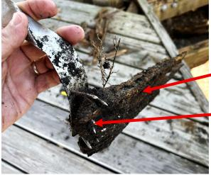
The wood member buried in the soil and nailed to wind strapping to counter wind uplift forces.
