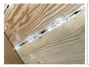
Unknown insects (or arachnids had left fibrous or web material between the preservative treated planks of the roof. These were wiped away to reveal no damage to the wood had occurred. This could be a maintenance issue to address with cleaning. The upper gazebo wood construction appeared to be in generally good condition and would be considered to have a long remaining useful life.
