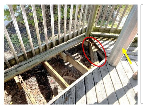
This photo shows the main gazebo columns (yellow arrow at the right side of the photo) that extend down and connect with the concrete piers in the lakebed. The deck planks placed in different directions to the interior deck planks as well as the supporting framing must rely on irregular directions and odd joist configurations and connections. (This is seen within the red ellipse located left of the main column.)
